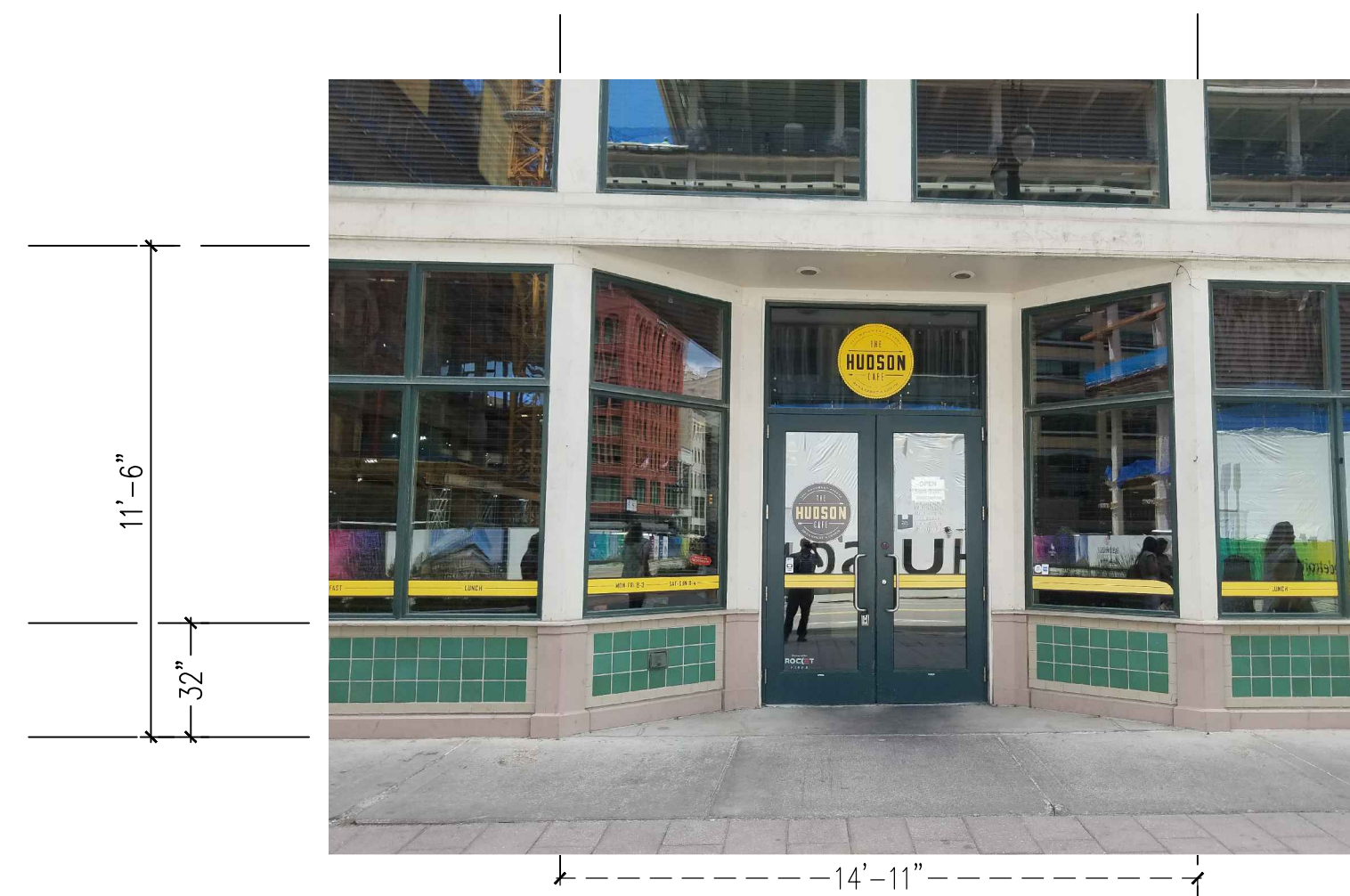
EXISTING FACE FRONT
