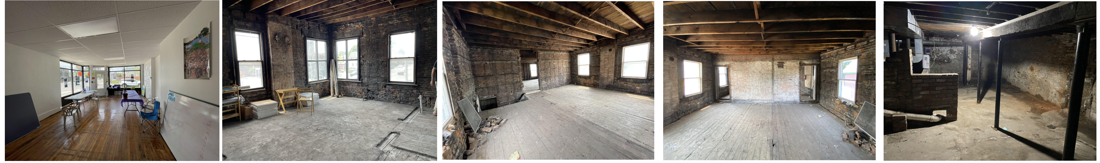
EXISTING CONDITIONS PHOTOS
