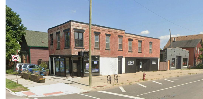
EXISTING CONDITIONS PHOTOS
