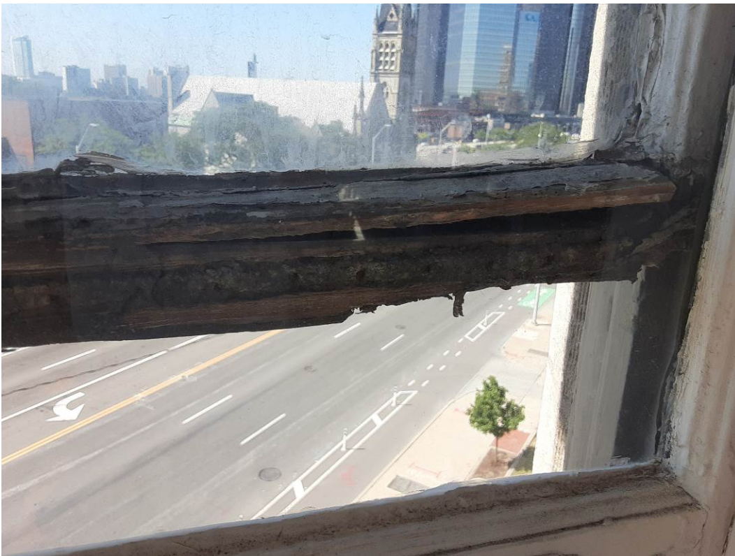
16. Typical interior meeting rail condition.
