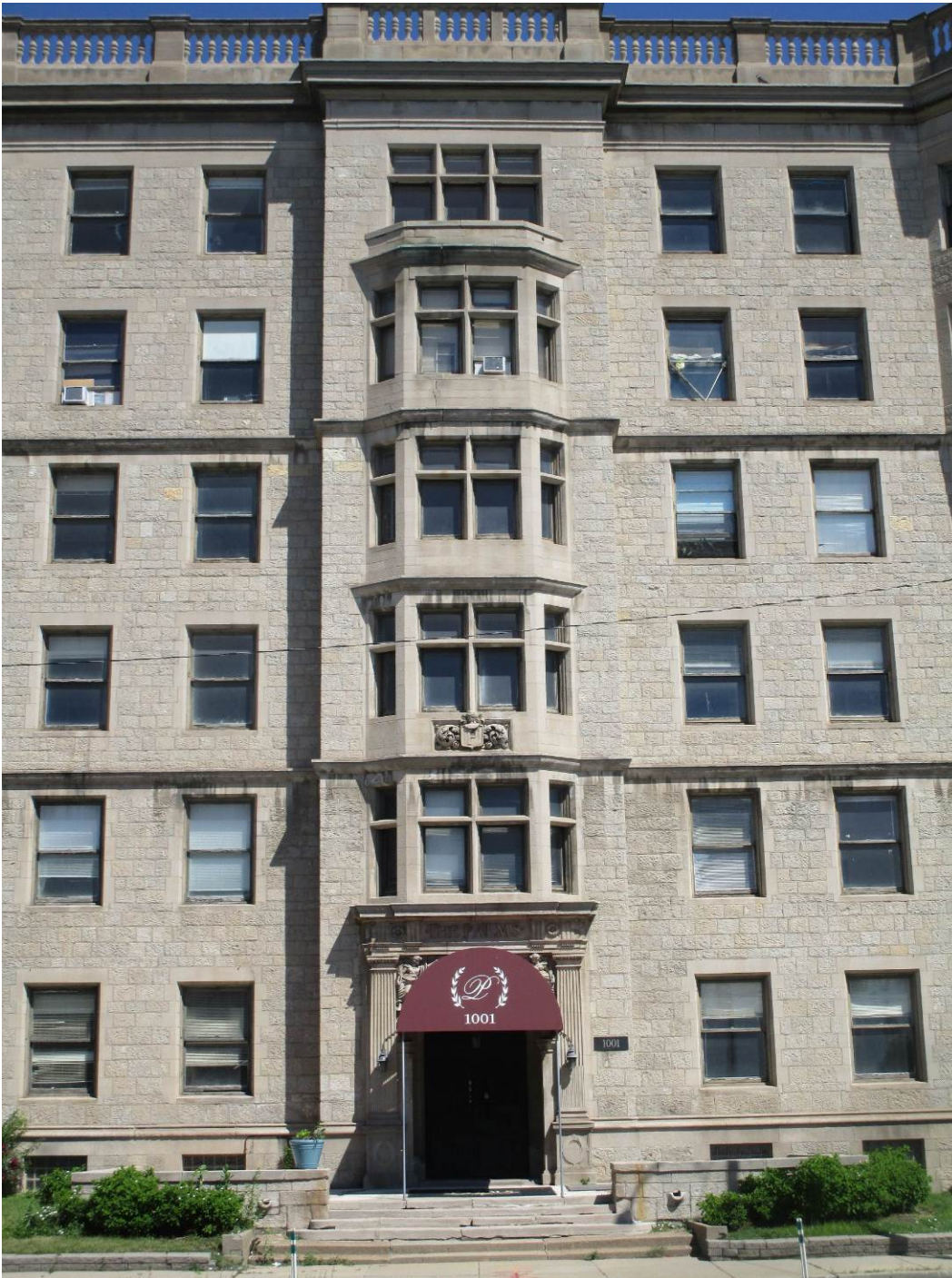
5. Partial South Elevation looking at main entry and terrace.
