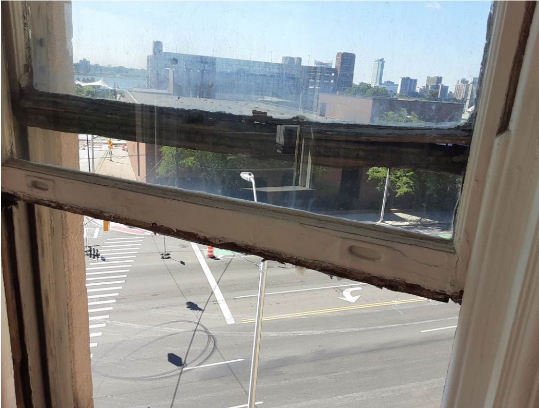
15. Typical interior meeting rail condition.
