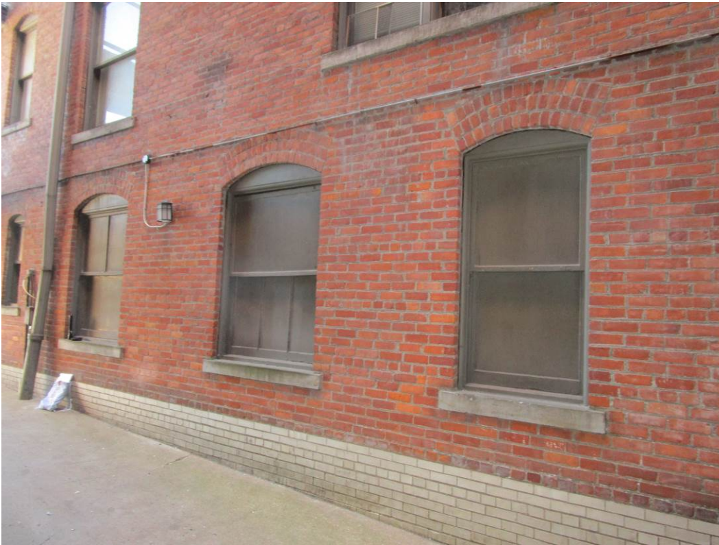
13. Typical wood double hung window in courtyard.
