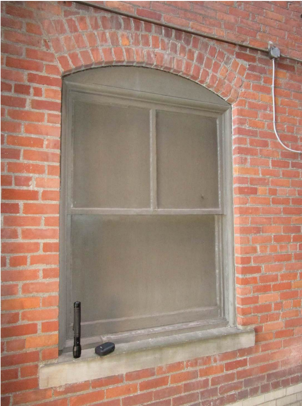
12. Typical wood double hung window in courtyard.
