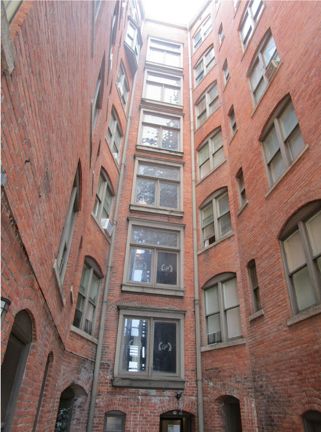
12. North Elevation in courtyard looking south at stair landing bay windows.
