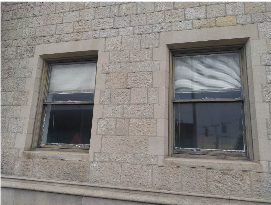
3. Typical double hung window at stone.
