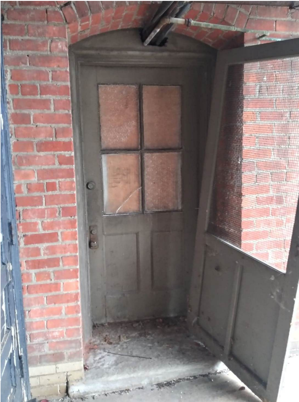
21. Typical existing fire escape door and screen in courtyard.
