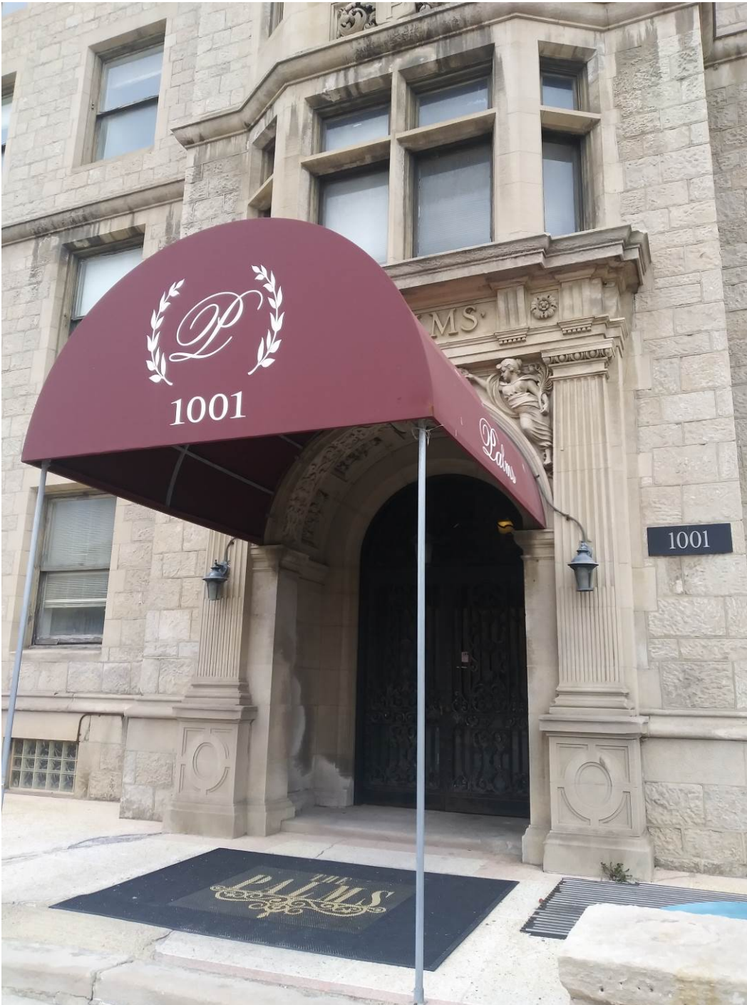
6. Main entry looking north.
