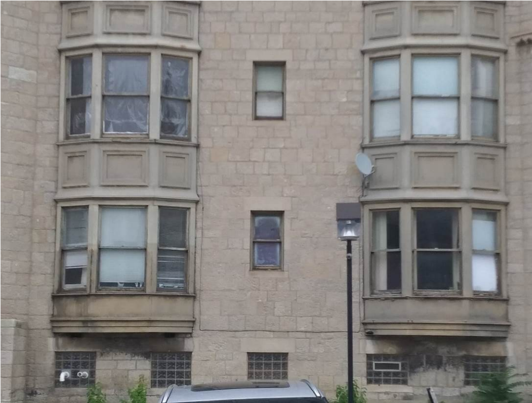
17. West Elevation looking east at bay windows (lower).
