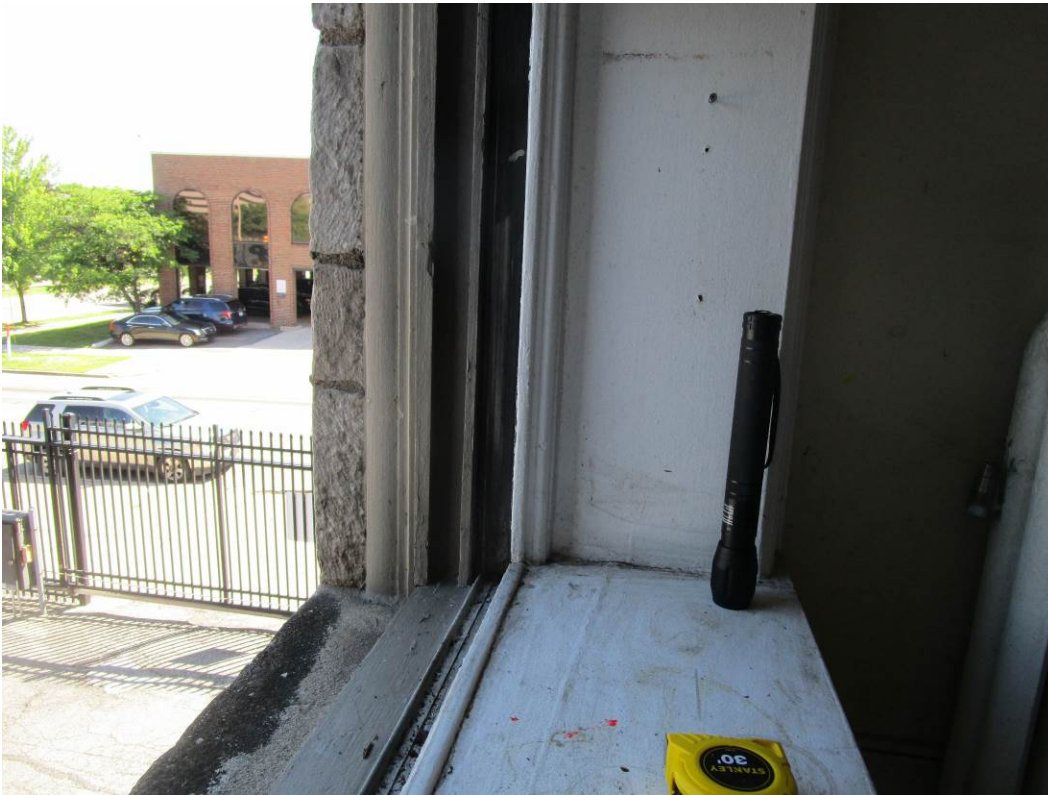
17. Typical interior sill condition.
