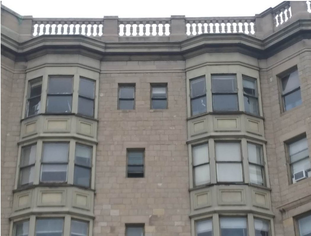
15. West Elevation looking east at bay windows (upper).
