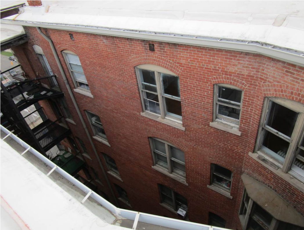
10. West Elevation in courtyard looking northeast.
