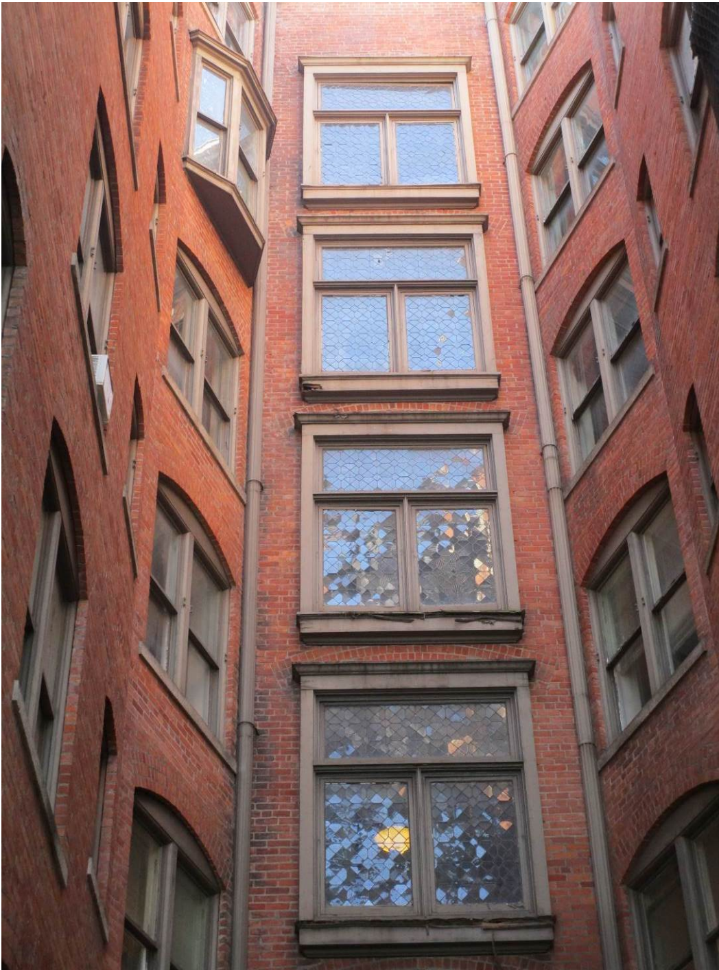
8. Courtyard north elevation, bay window at stair landing with stained glass to be restored (upper).
