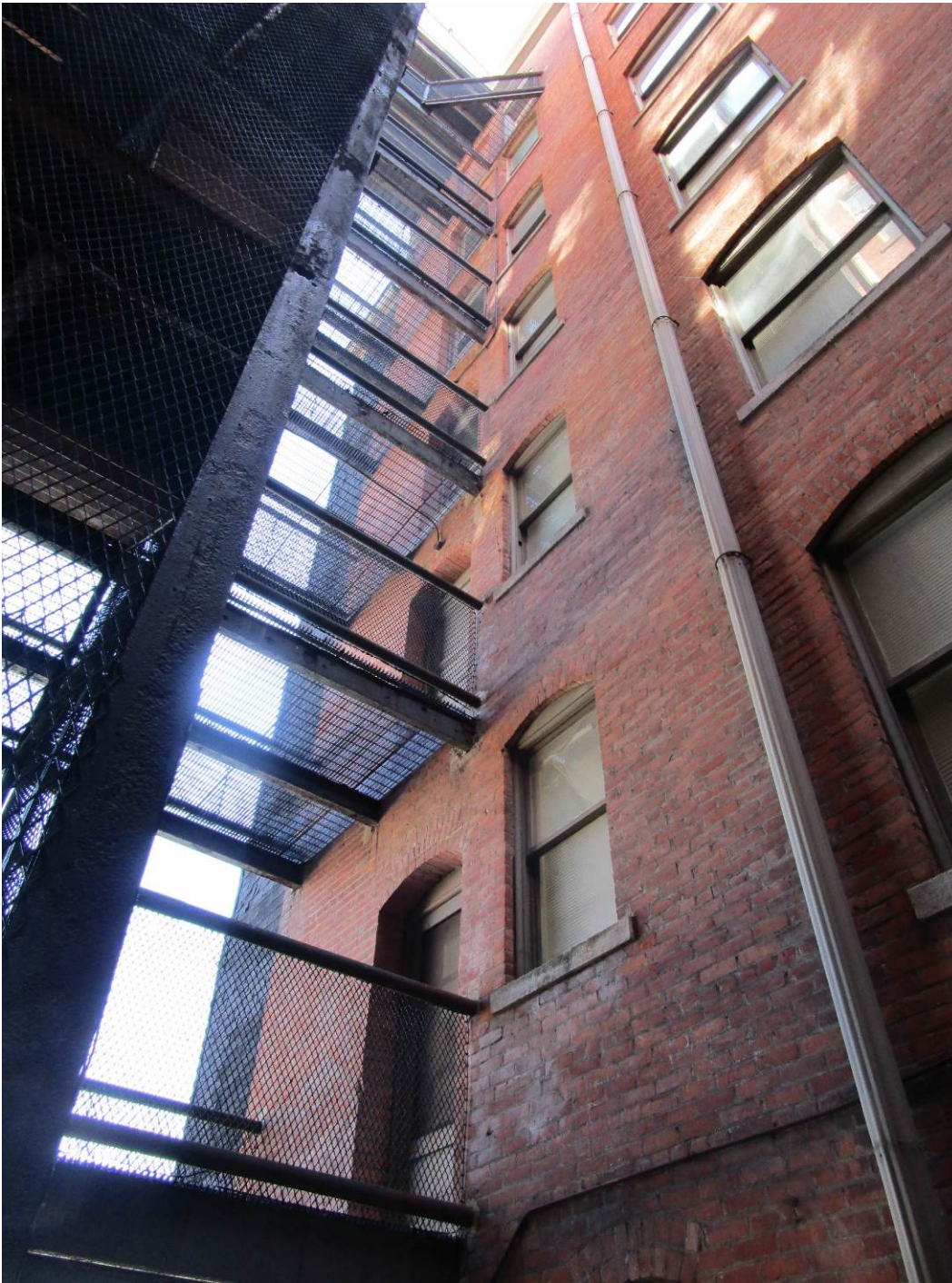
13. Northeast corner in courtyard looking northeast at fire escape.
