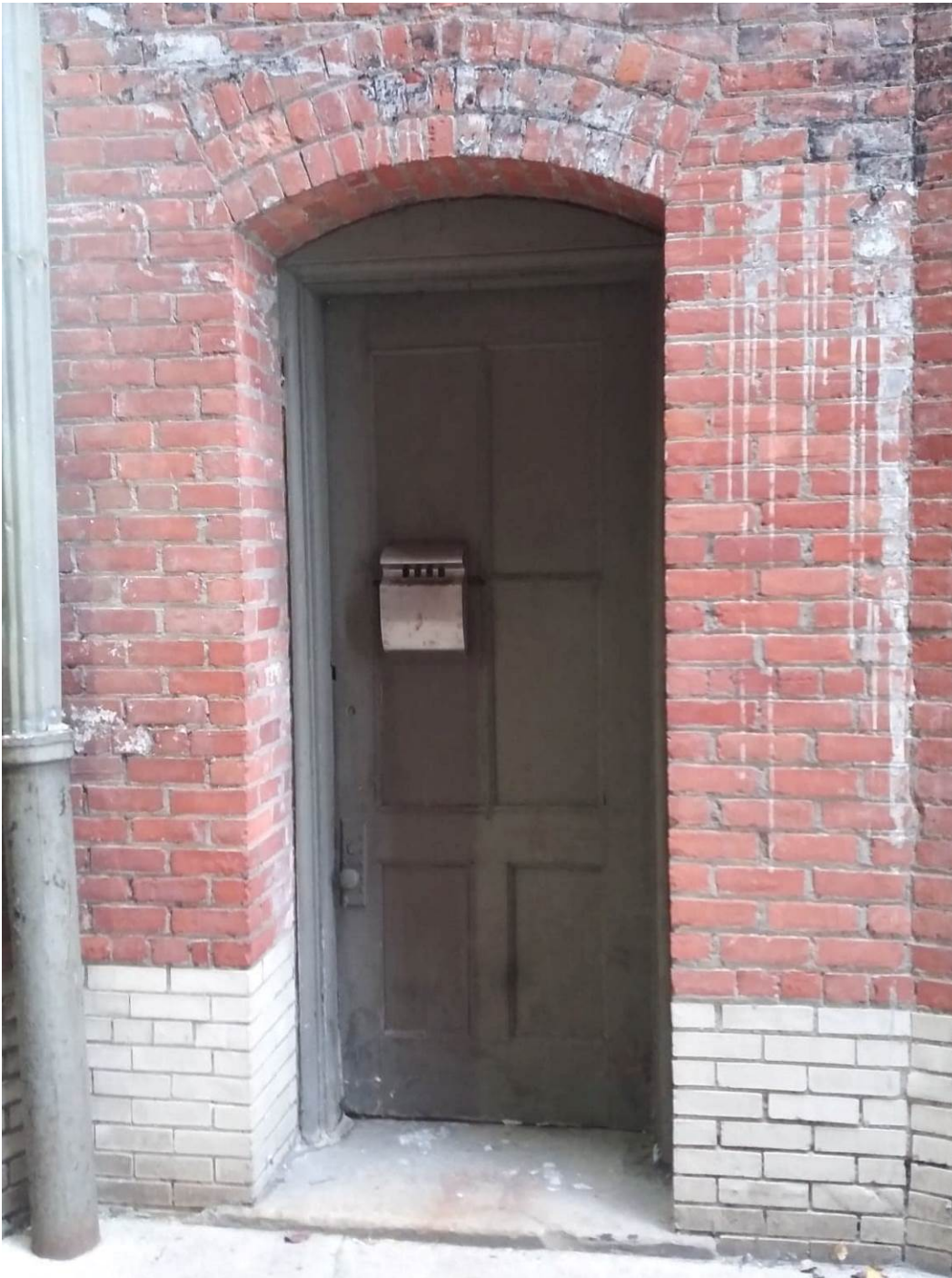
20. Existing door in southwest corner in courtyard.
