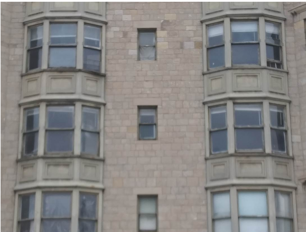
16. West Elevation looking east at bay windows (middle).
