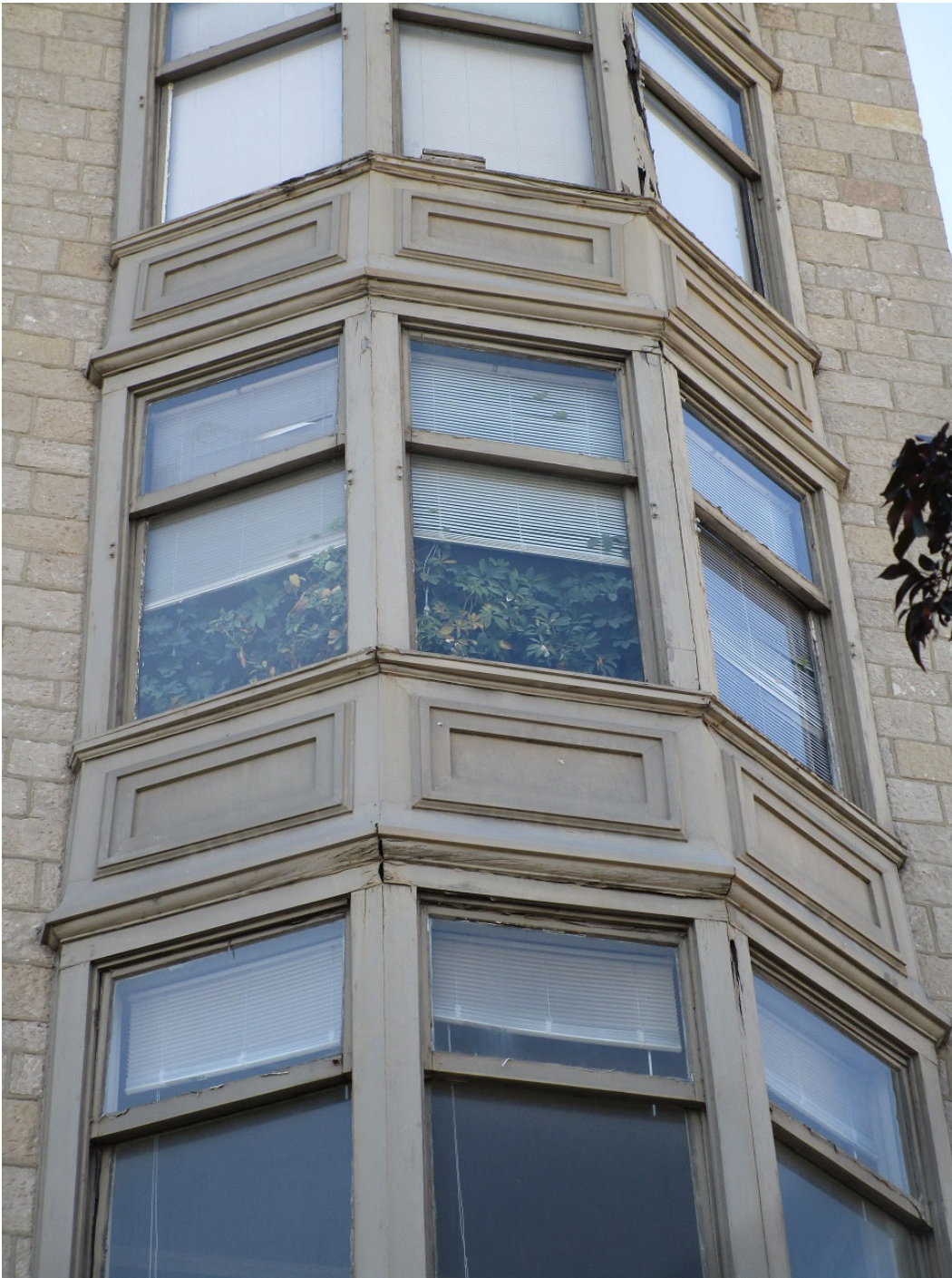
21. North Elevation looking south at bay window (middle).
