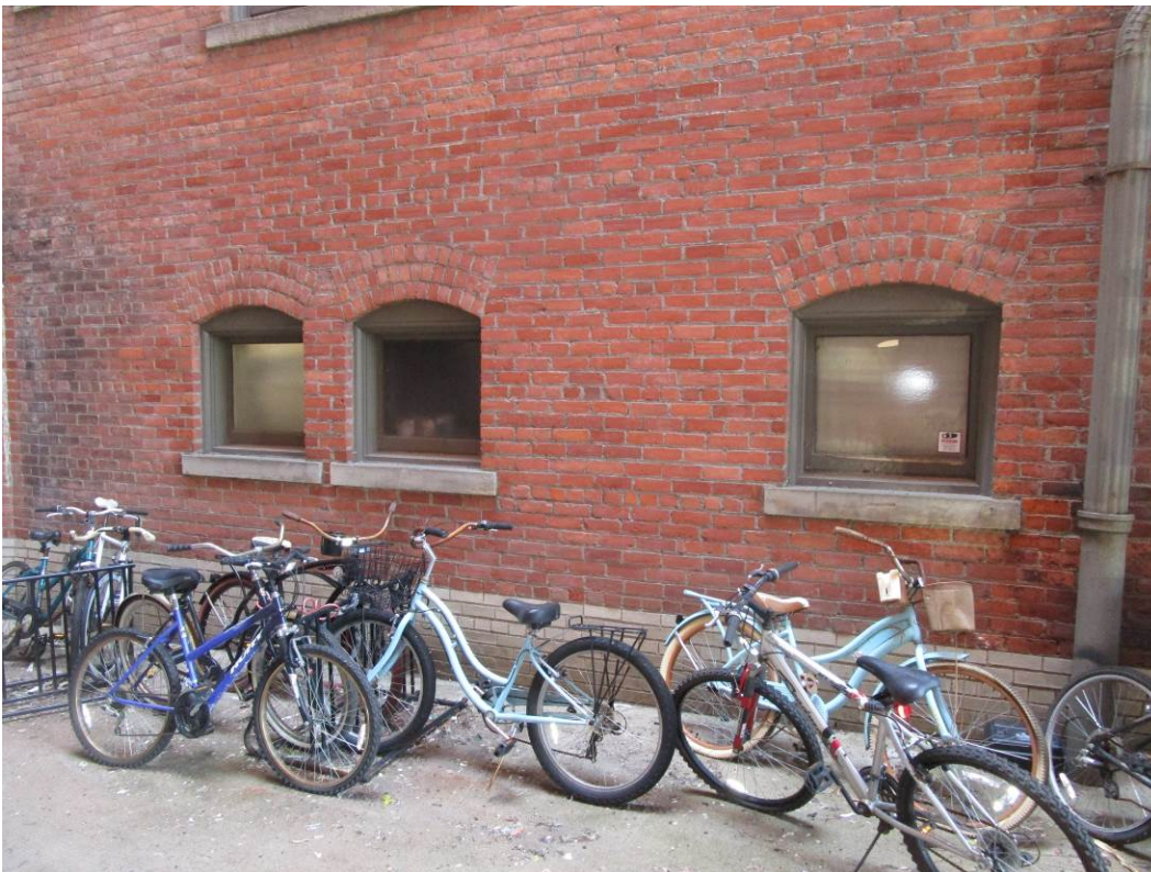
14. Typical wood awning window in courtyard looking west.
