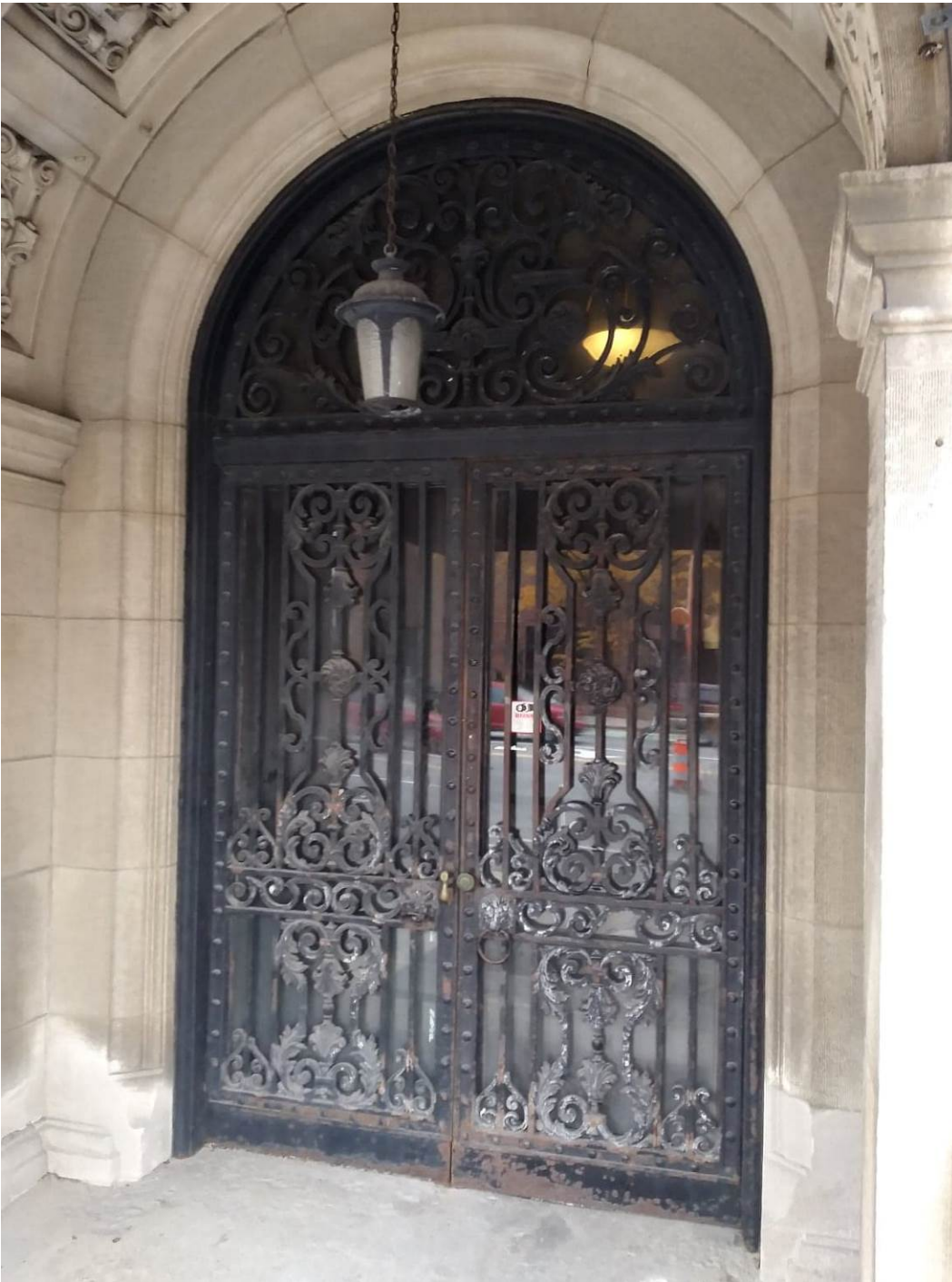
7. Main entry looking north at steel entry gate.
