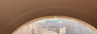
Semi circular window 2. Original was stolen. We replaced it with a glass pane. Note: chipping lead paint, and cracked wall under the window due to water damage.
