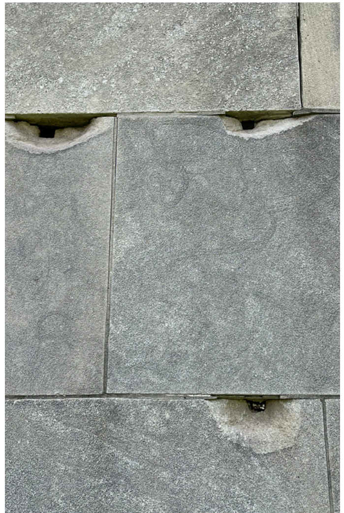
Detail of Masonry, 2022
