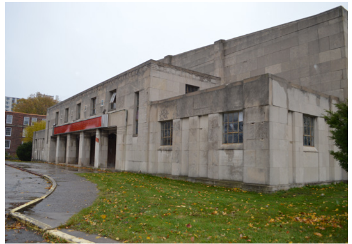
Primary facade of the Brodhead Naval Armory, 2022
