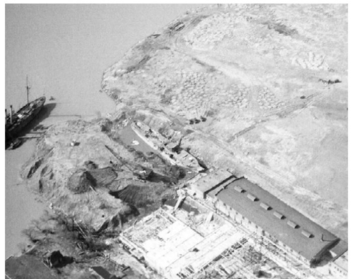
Brodhead Naval Armory, under construction
