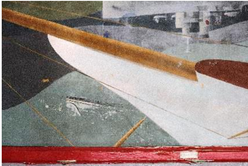
Detail of a repainted area along the bottom of mural. The overpaint is flaking and has exposed some of the earlier design.
