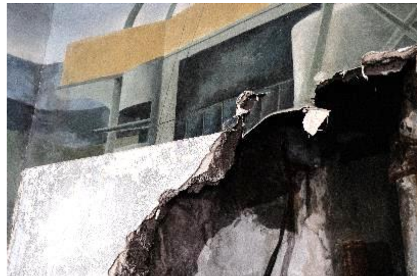
Closer detail of the canvas loss. It also shows the loose edges of the remaining canvas.
