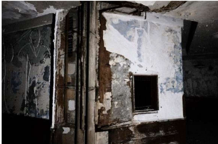
Detail of the eastern wall where relief panel has been removed.
