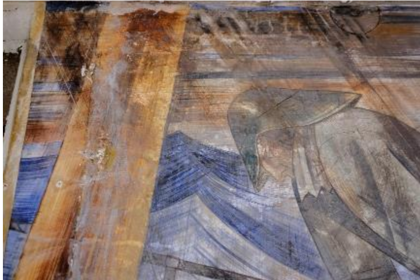
Detail Photo showing the water damage on the upper left corner of the mural. It has caused some losses, surface discoloration and blanching.
