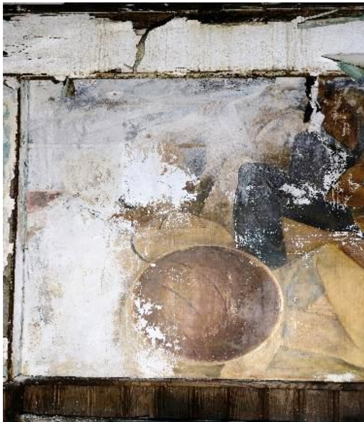
Detail of the left-hand portion of the fresco. Water damage has caused significant damage and loss.
