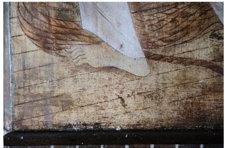
Detail showing heavy blanching, discoloration and dark marks.
