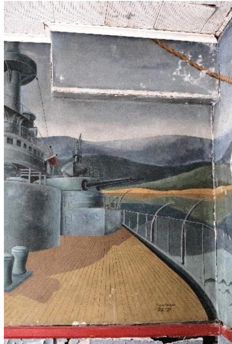
Detail of the right hand side of the mural. The small portion of canvas on the bump out and the entire section of below has delaminated and is loose.
