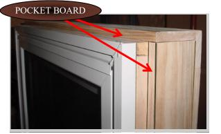
Classic Fit has a pocket board on the main frame. The pocket board is found on both jambs and the header, but not on the sill.
