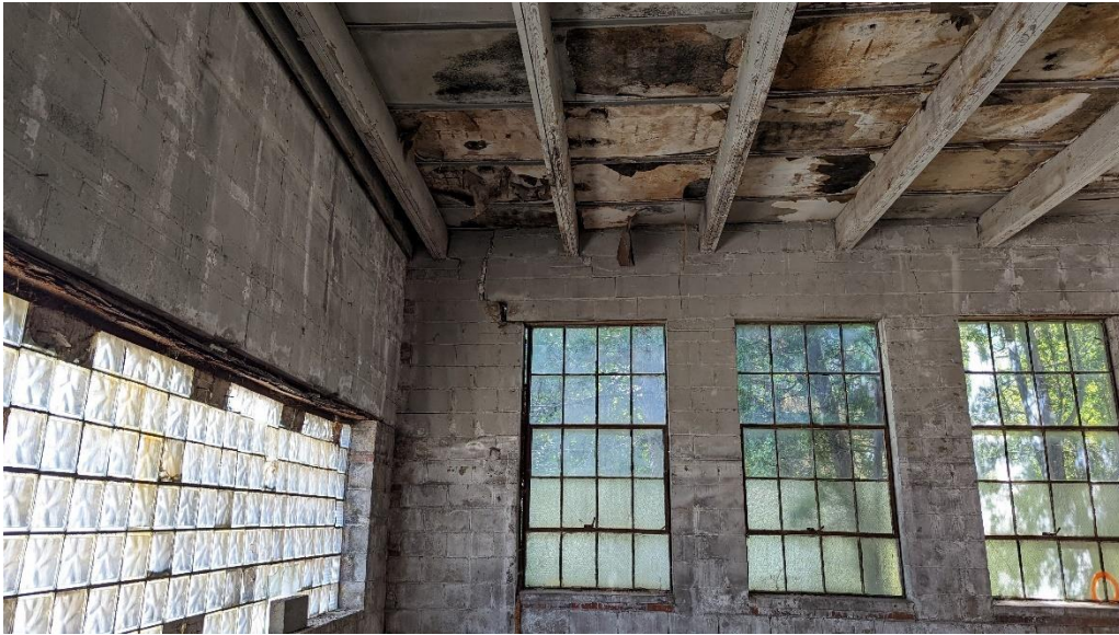
Picture A. 7: Interior View of the South Addition.
