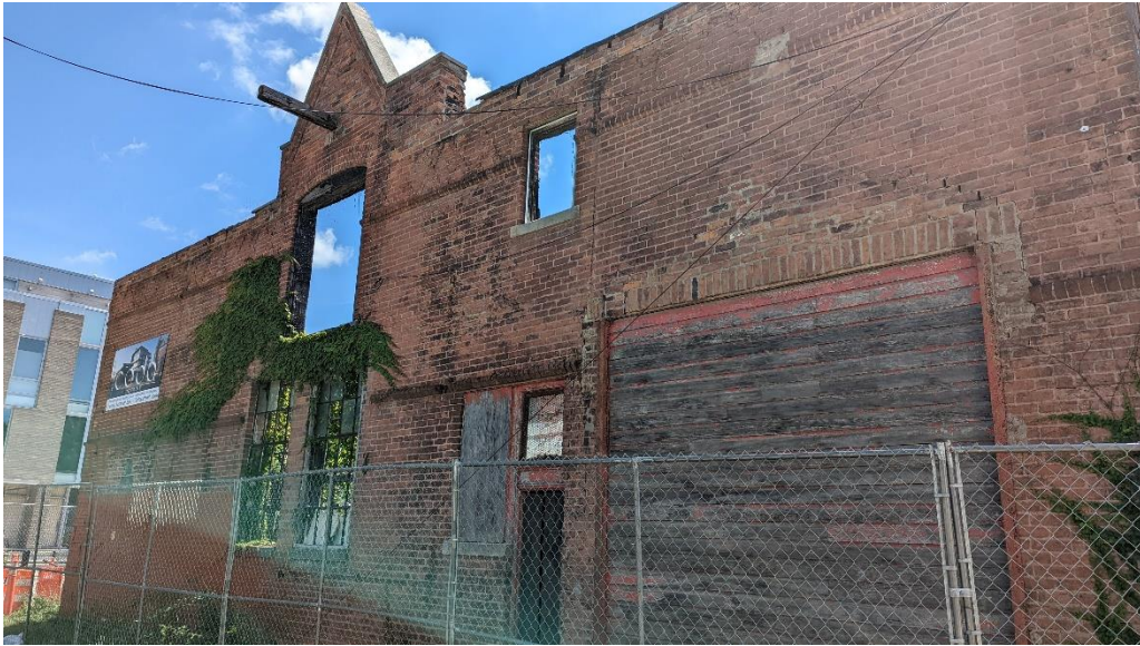
Picture A. 5: Exterior View of North Wall.
