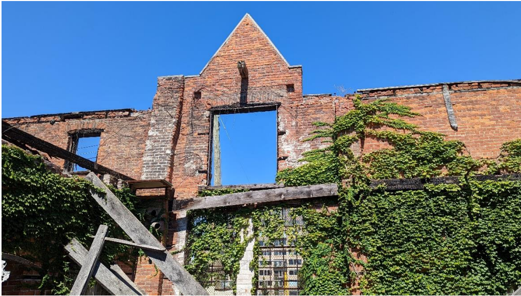
Picture A. 3: View of North Wall.
