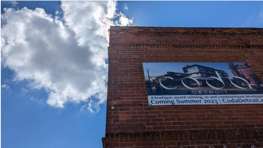
Picture 12: Crack Along Intersection of Walls at Northeast Corner.
