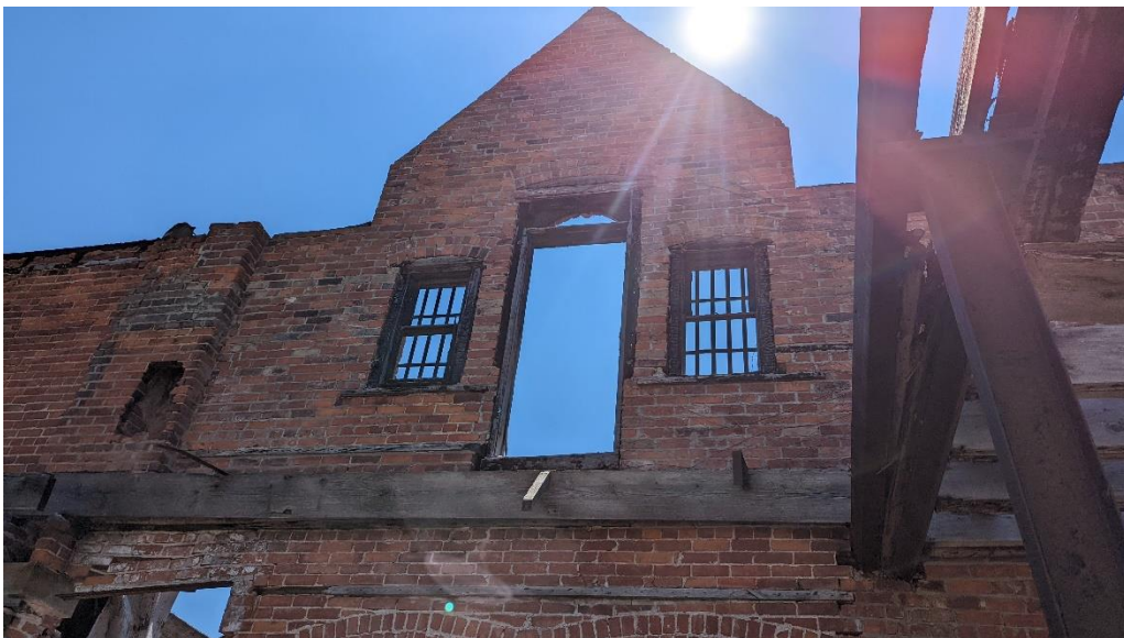
Picture 10: View of South Wall with Non Square Openings
