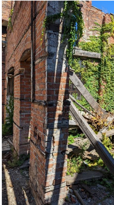
Picture 17: Wall in Center of Building.
