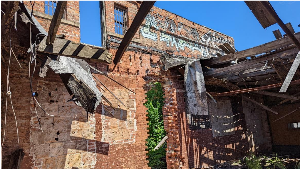
Picture A. 1: View of South Wall.
