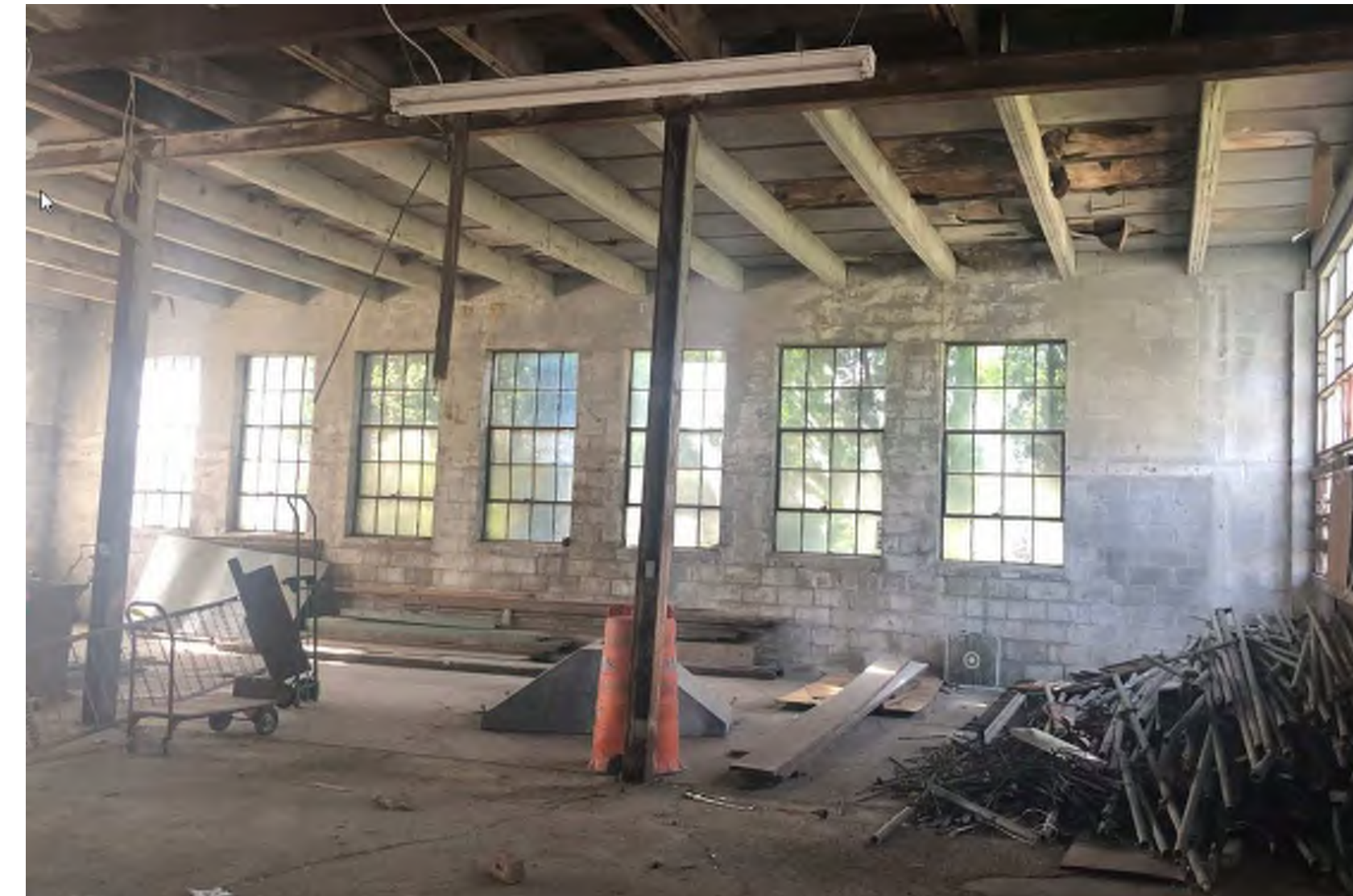
IMAGE OF WINDOWS TO BE SALVAGED, FROM BUILDING INTERIOR
