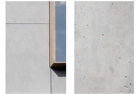
CAST-IN-PLACE ARCHITECTURAL CONCRETE FOUNDATION WALLS
