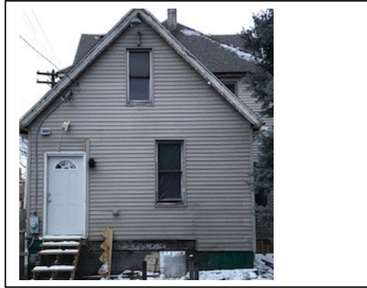
west side of house – Back yard
