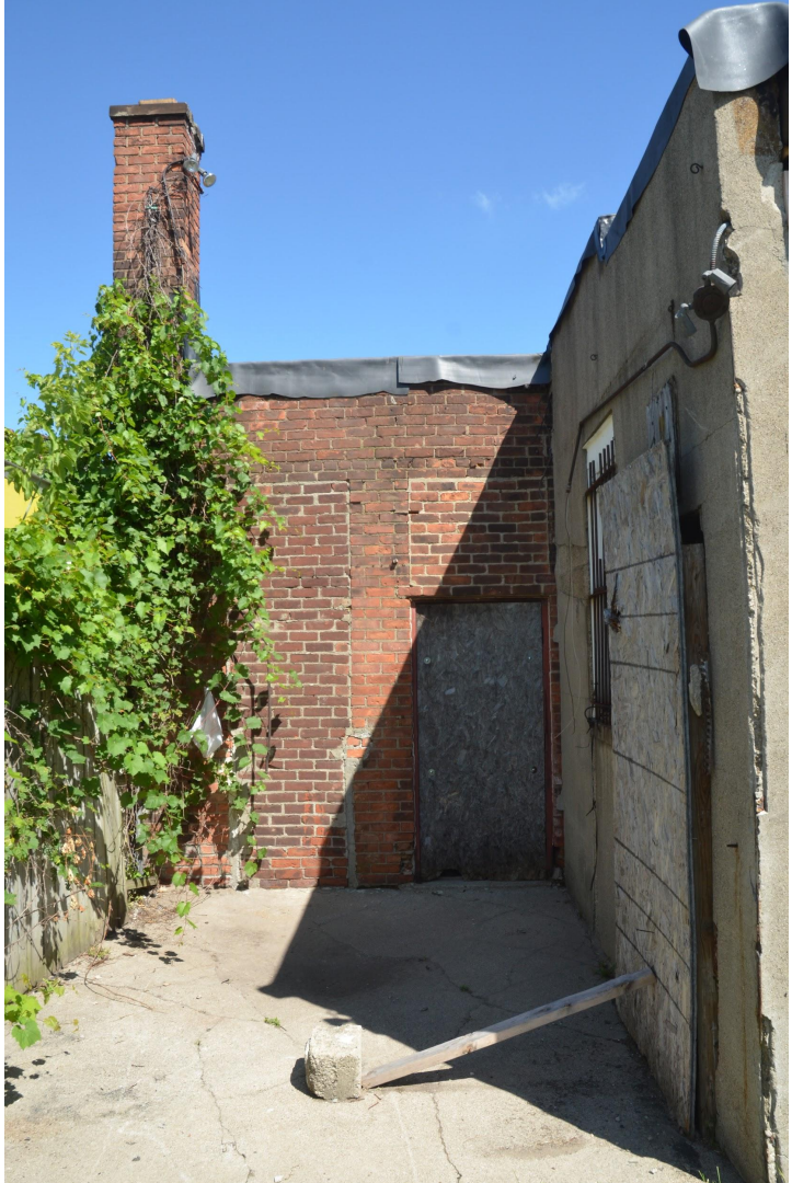
Blue Bird Inn Rear Doors and Gutters
