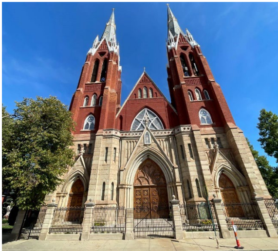
Front of Church (West)
