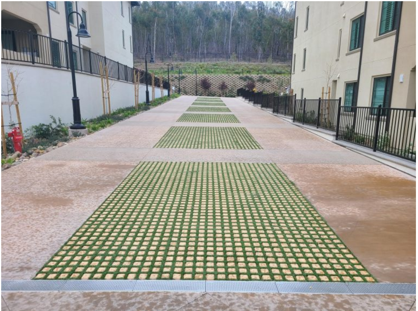
Fire Lane – Drivable Grass® with Pre-Cut Turf Infill
