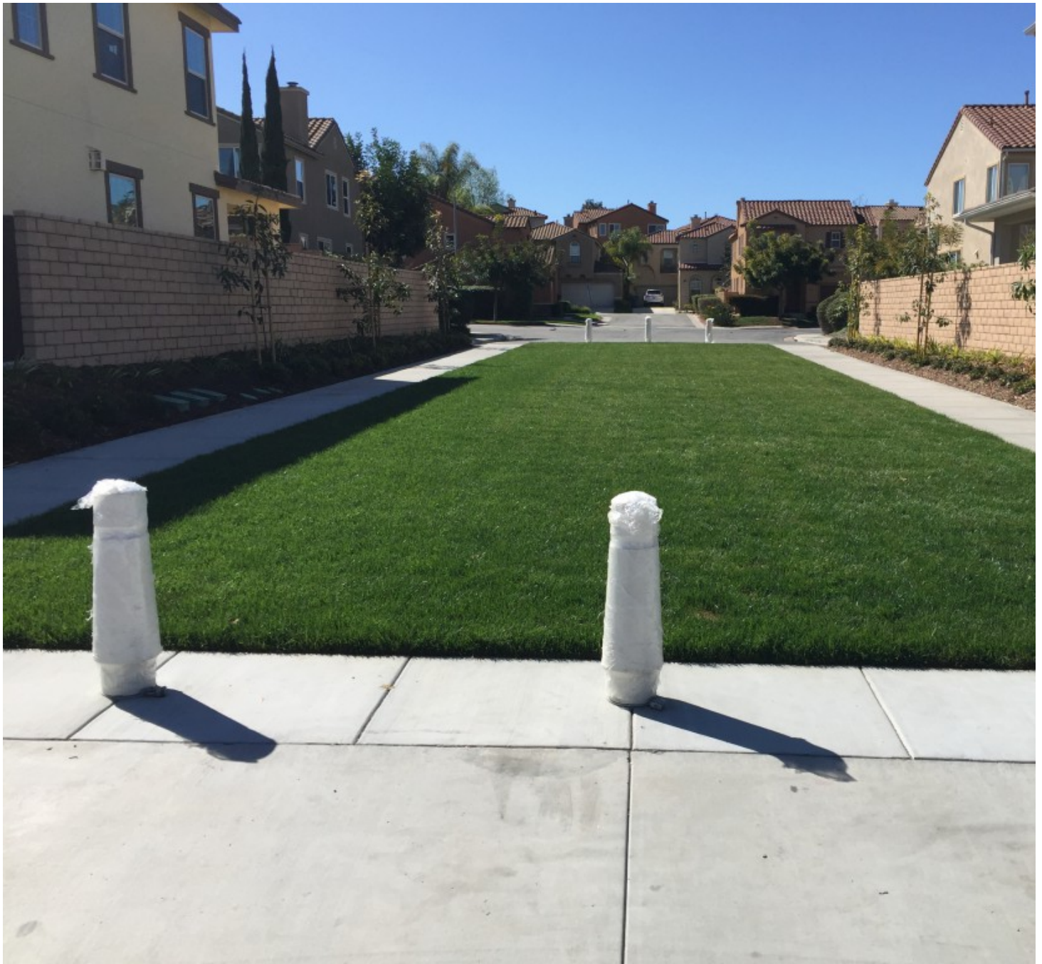
Fire Lane – Drivable Grass® With Planted Infill
