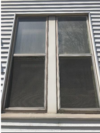
2 windows to be replaced on southeast side of house facing southeast
