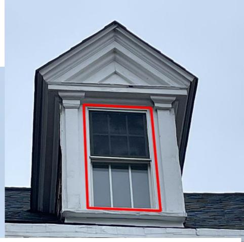
Proposed window units will be installed inside of the wood trim/brickmould and the existing wood trim/brickmould will not be covered with aluminum nor will it be removed or disturbed.
