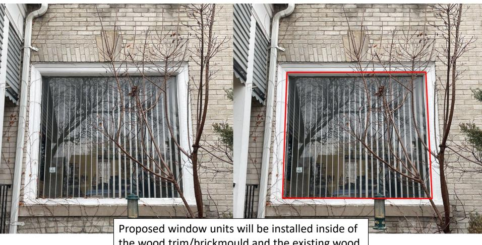
the wood trim/brickmould and the existing wood trim/brickmould will not be covered with aluminum nor will it be removed or disturbed.
