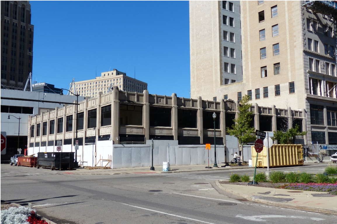
Figure #1: Exterior, East and South Facades, Description, Looking Northwest. 10/16/17.
