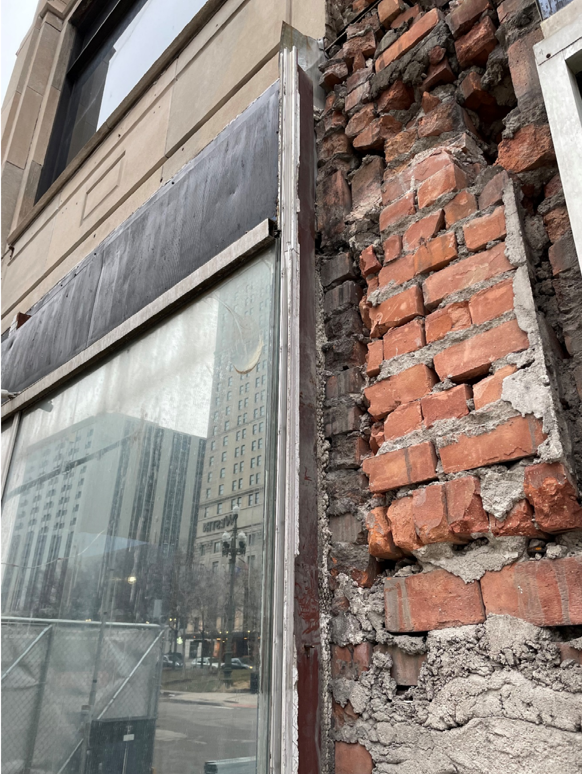
Figure #7: Exterior, East Façade Storefront Connection. 04/05/22.
