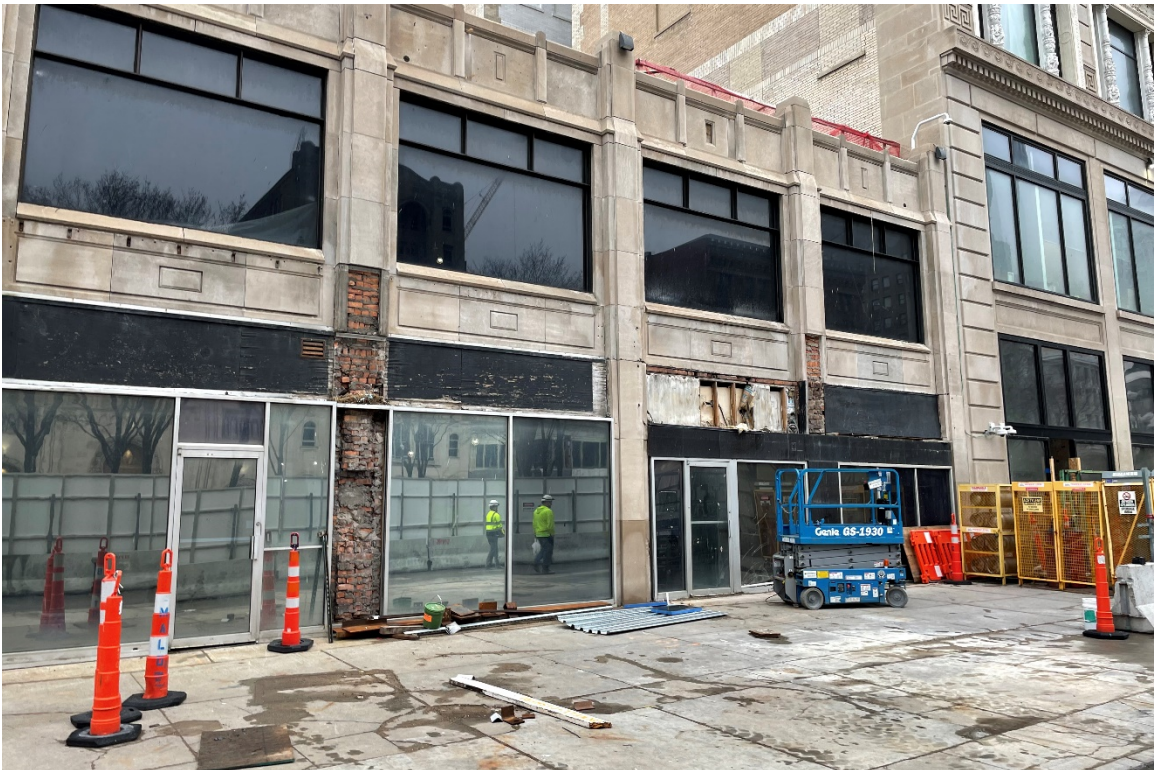
Figure #2: Exterior, East Facade, Looking North. 04/05/22.
