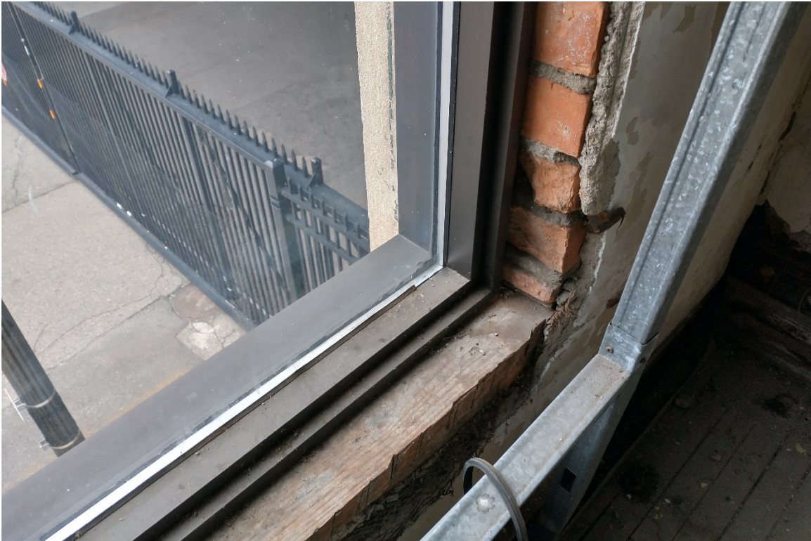
Figure #16: 2 nd Floor, Storefront Sill. 10/30/20.
