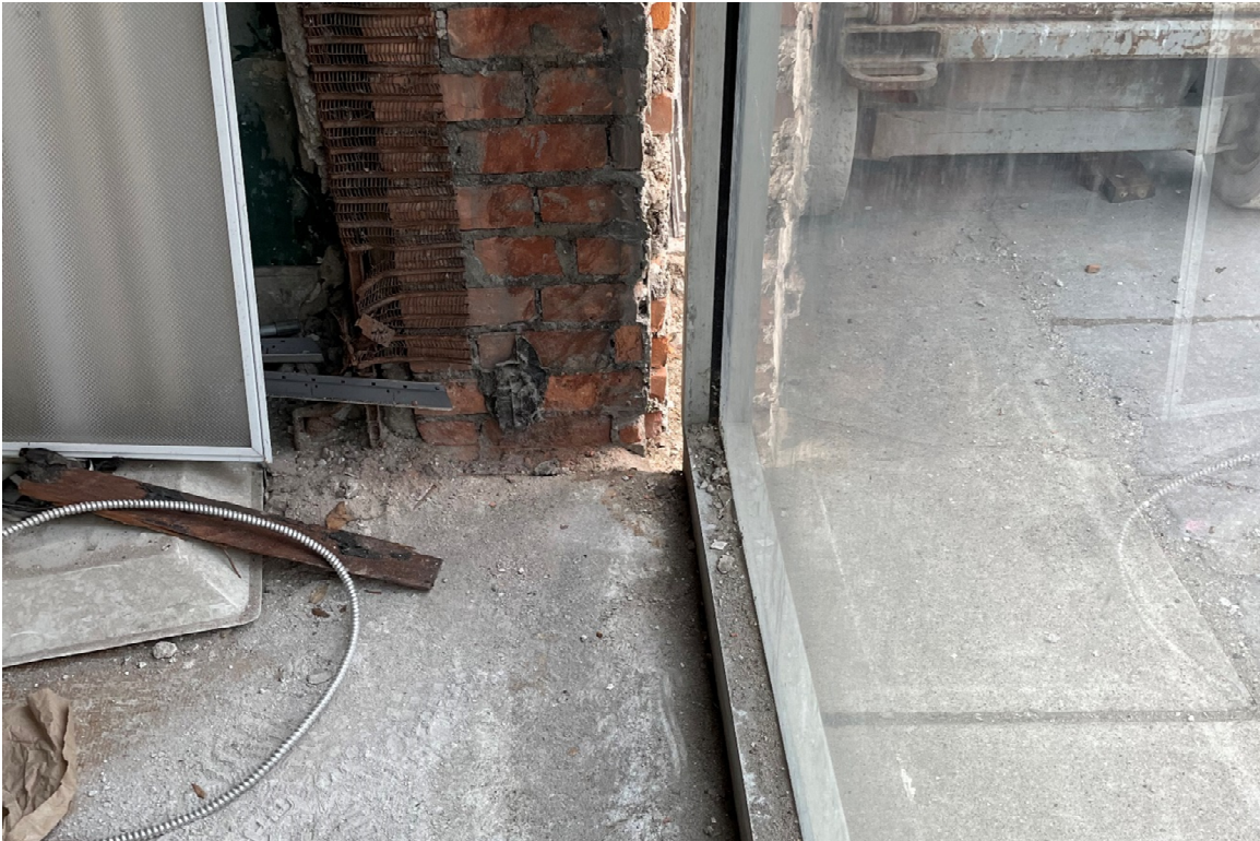
Figure #12: 1 st Floor, Storefront Sill. 04/01/22.
