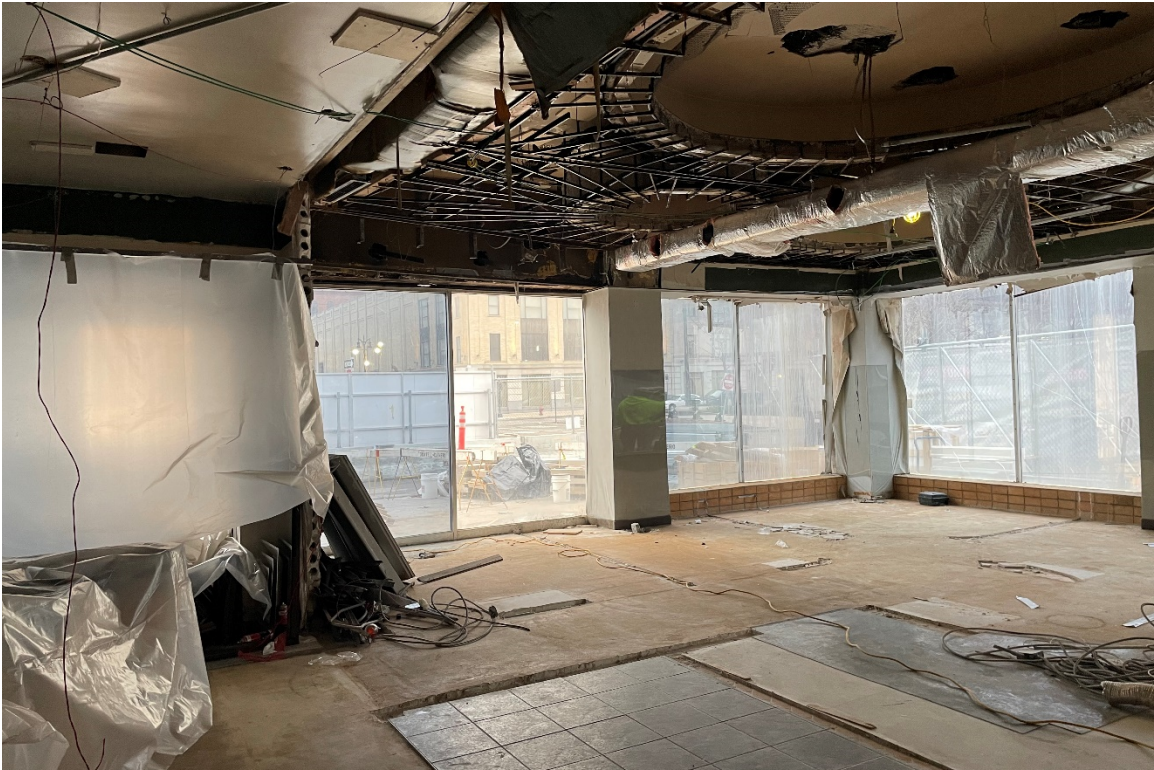
Figure #8: 1 st Floor, Southeast Storefront, Looking Southeast. 04/05/22.
