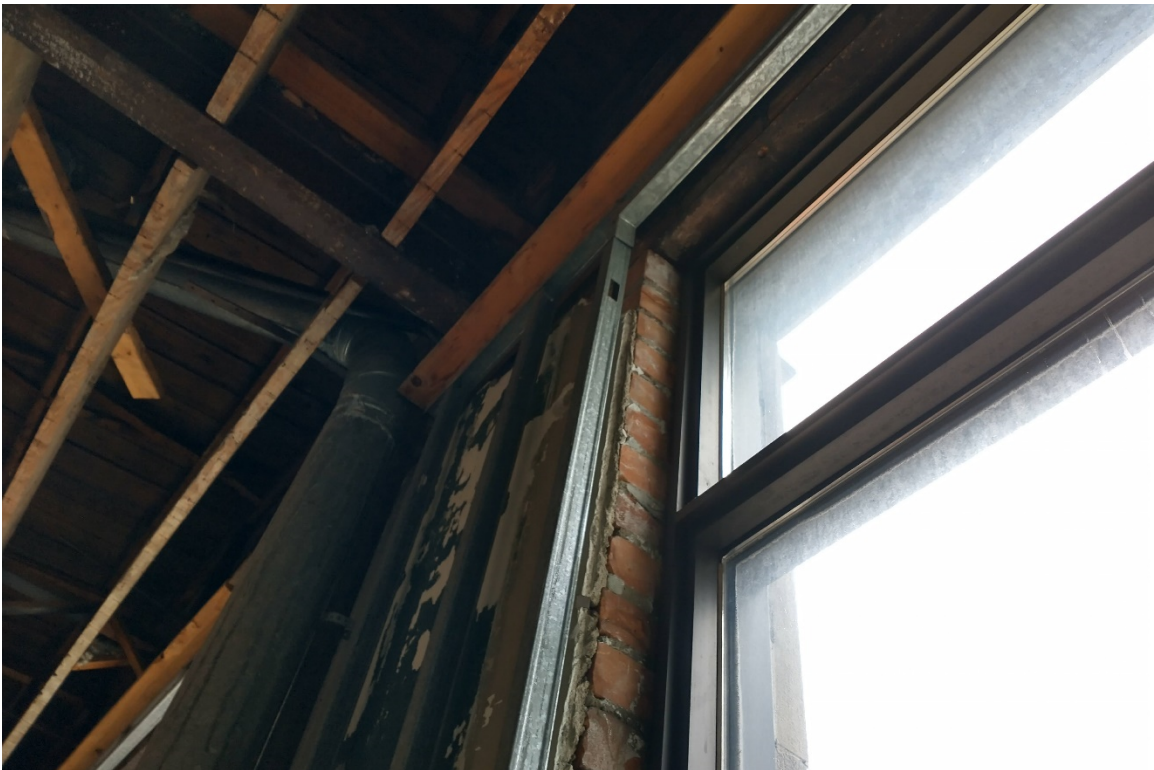
Figure #17: 2 nd Floor, Storefront Header. 10/30/20.
