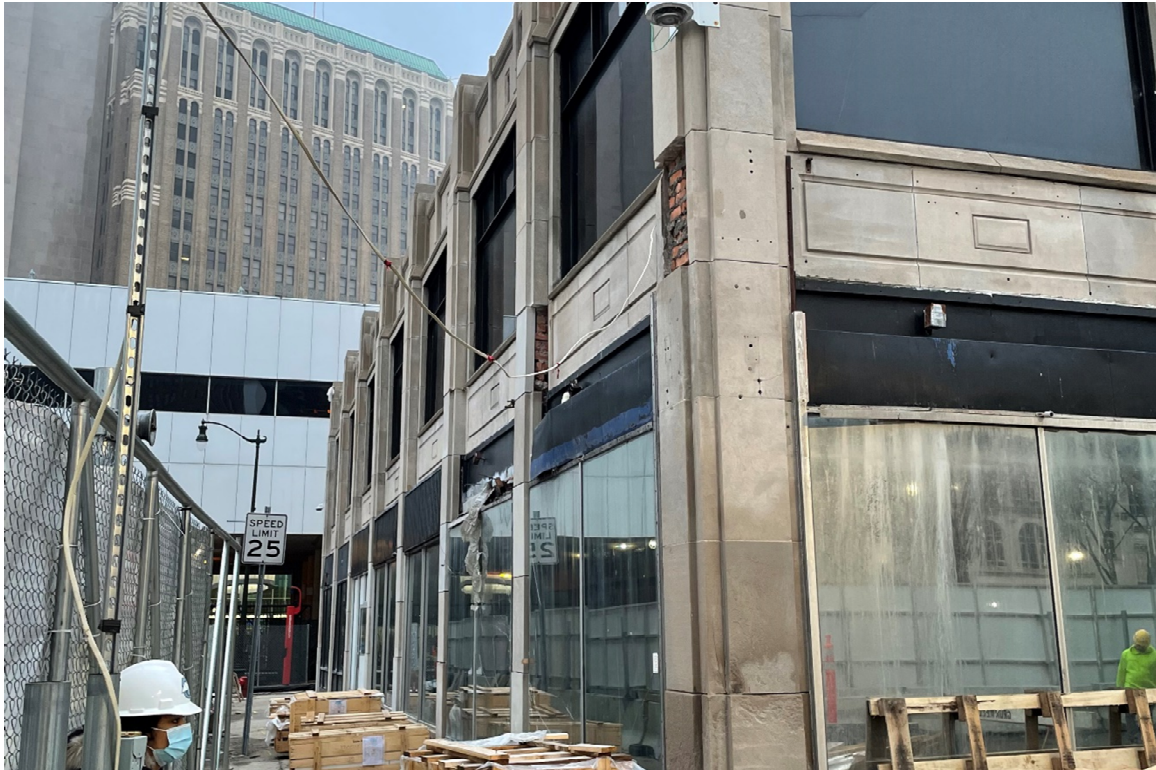
Figure #5: Exterior, South Facade, Looking South. 04/05/22.
