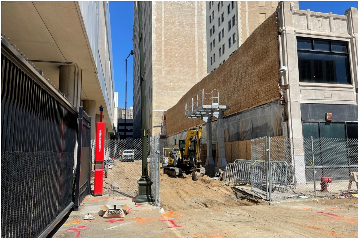
Figure #6: Exterior, West Facade, Looking North. 04/12/22.
