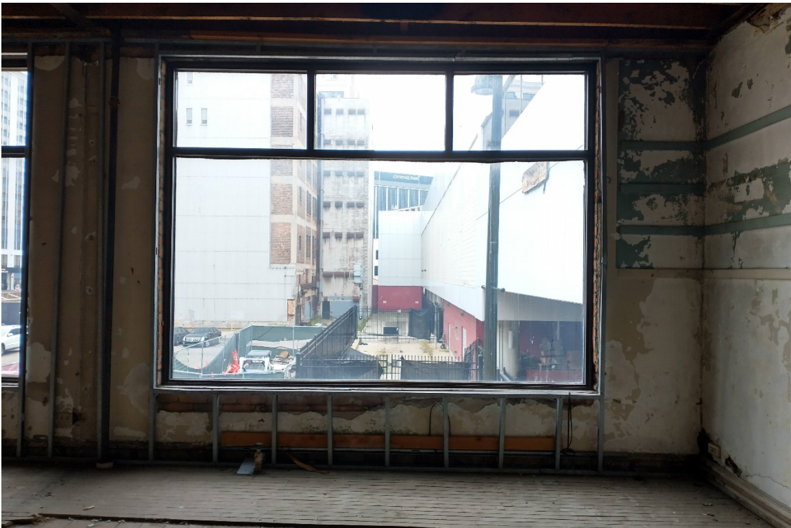
Figure #15: 2 nd Floor, Storefront, Looking South. 10/30/20.
