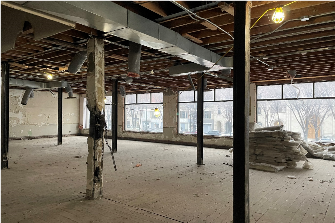
Figure #14: 2 nd Floor, East Storefront, Looking Northeast. 04/05/22.
