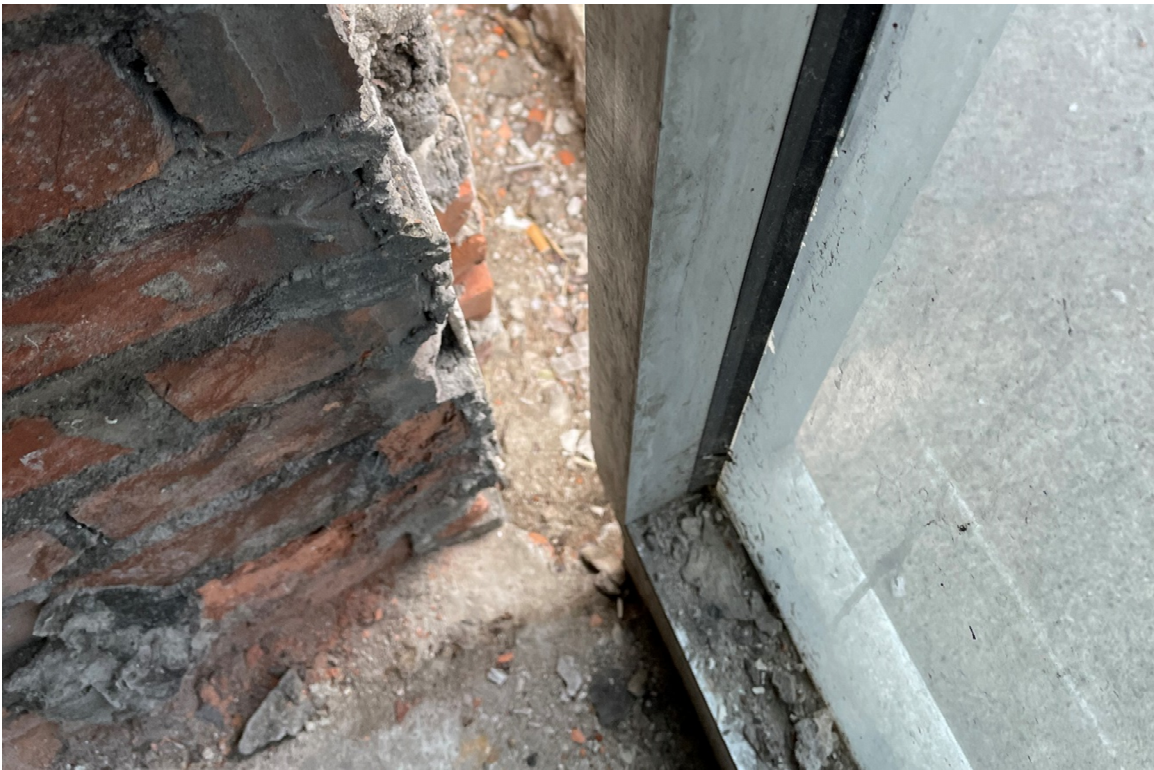
Figure #13: 1 st Floor, Storefront Sill. 04/01/22.
