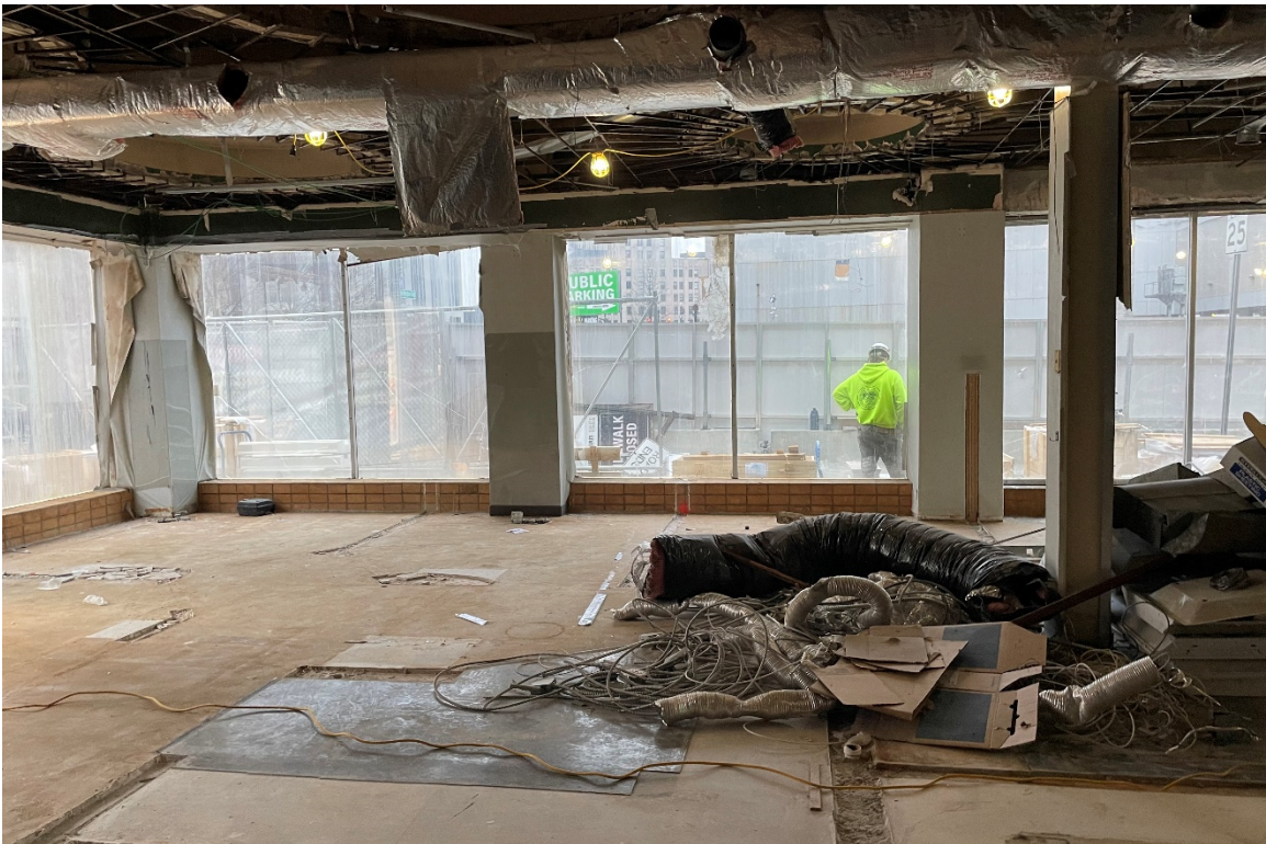
Figure #9: 1 st Floor, South Storefront, Looking South. 04/05/22.
