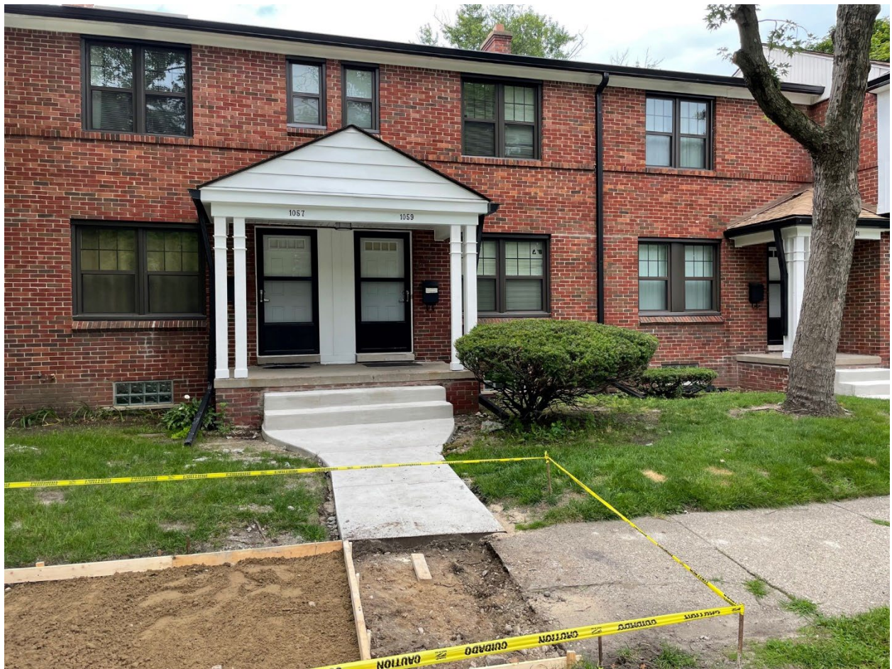
Photo 4: Phot showing new windows
