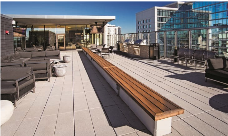
All Photos: Catalyst, Chicago, IL; Owner: Marquette Companies, Architect: Brininstool + Lynch; Landscape Architect: Latlin Design Group; Size & Color: 23 1/2" x 35 3/8" with score, Charcoal, Limestone Gray; Finish: Tudor®
