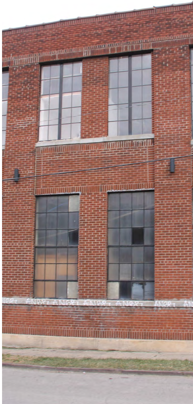
Example of Incorrect Replica of Steel Windows. Existing Original Window on 1st Floor. Incorrect Replication on 2nd Floor.
