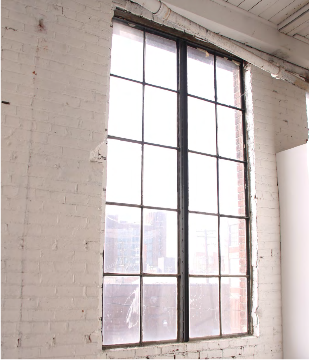
Interior View of Replica Steel Window
