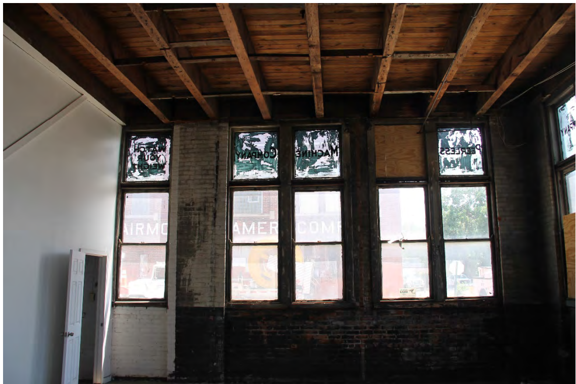
Interior View 1st Floor South Wall Partial
