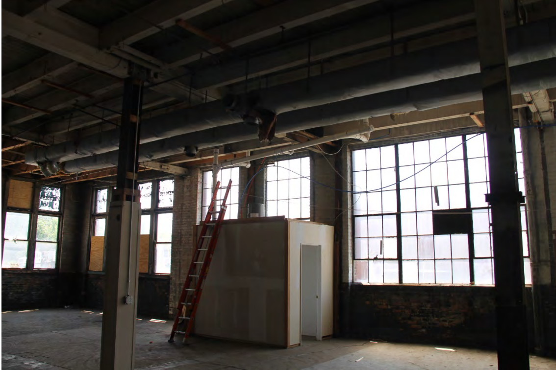
Interior View 1st Floor West Wall Partial, and South Wall Partial
