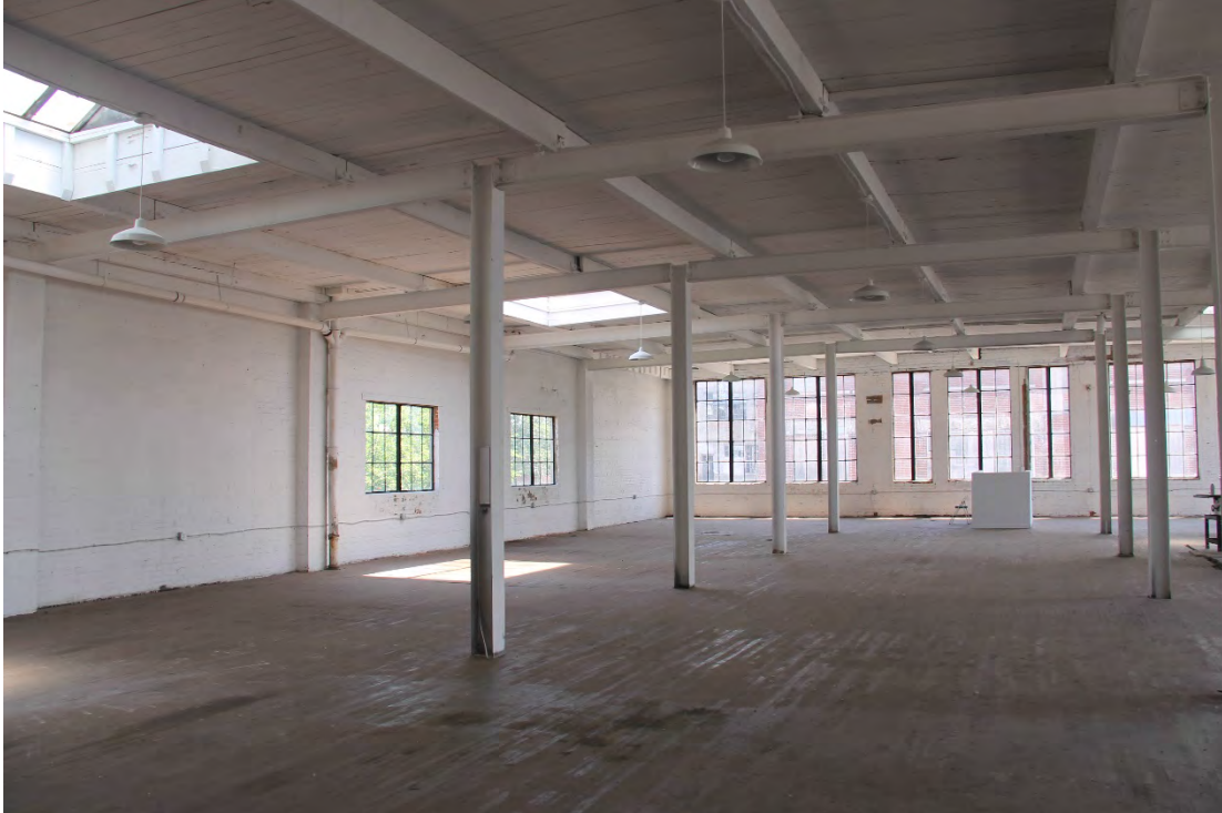
Interior View 2nd Floor East and South Walls
