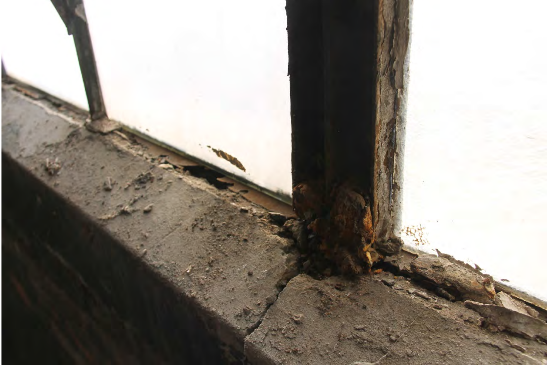
Typical Mullion and Bottom Rail Condition of Existing Steel Window, Interior View
