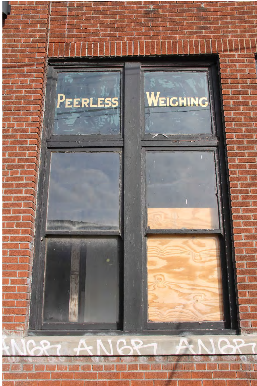
Exterior View of Typical Wood Double Hung
