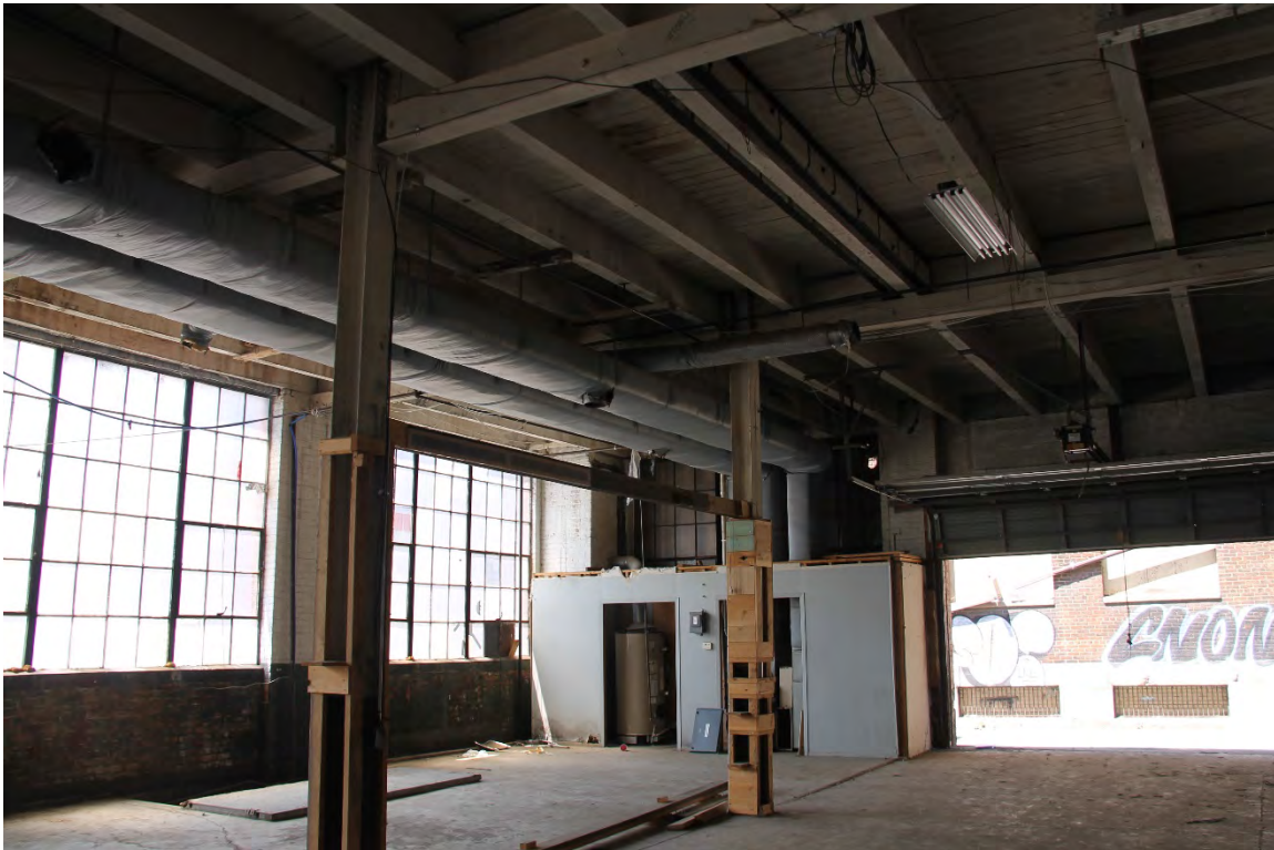
Interior View 1st Floor West Wall Partial, and North Wall Partial
