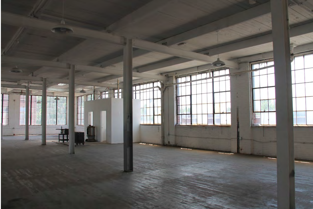
Interior View 2nd Floor West and South Walls
