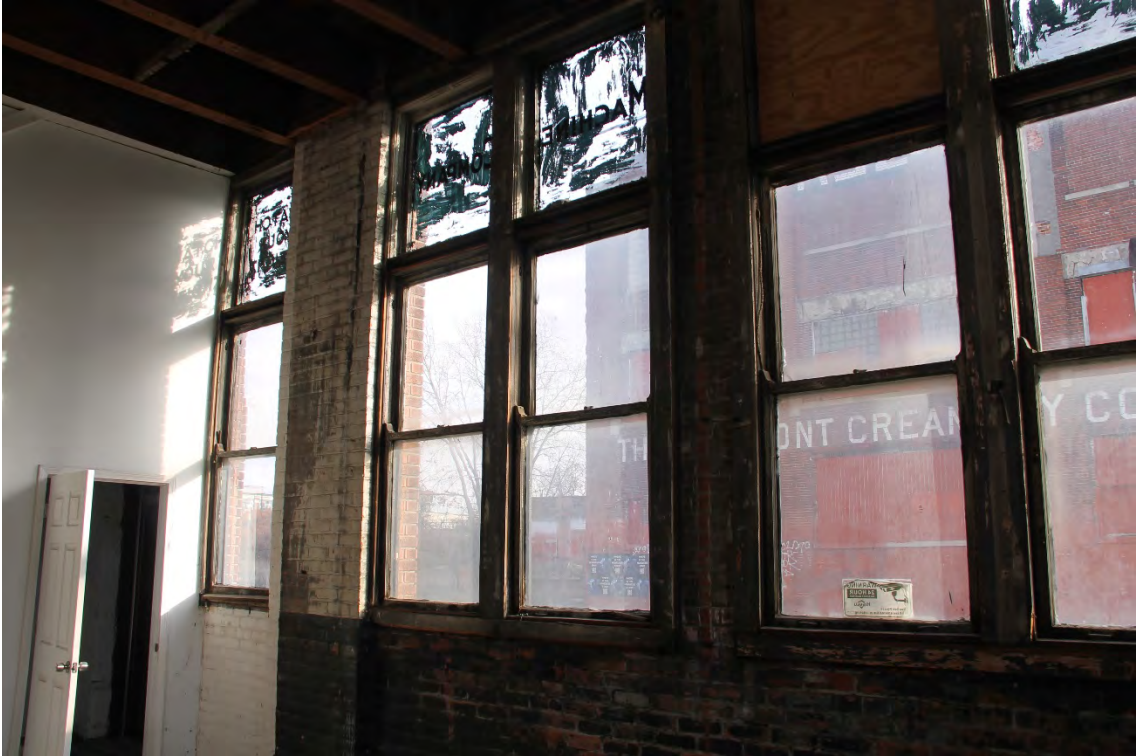
Interior View of Wood Double Hungs
