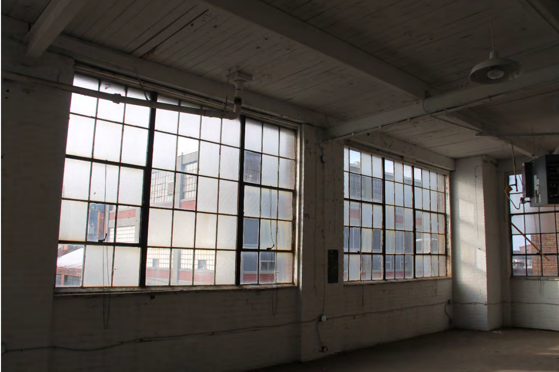
Interior of Typical Original Steel Windows
