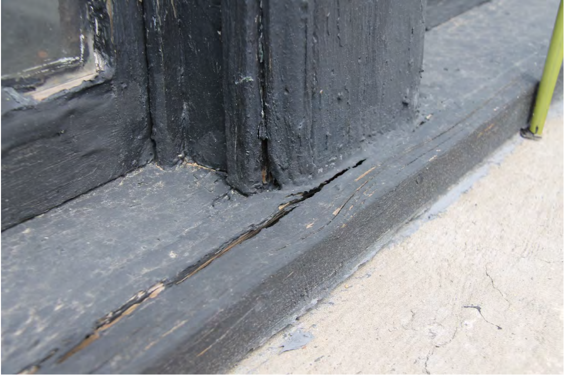
Exterior View of Split Sill
