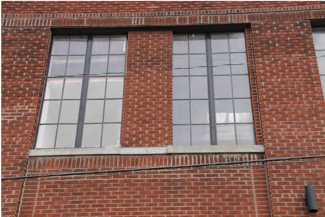
Exterior of Replica Steel Windows
