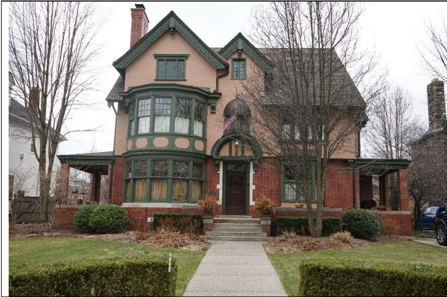
Photo 1 Front of house from Burns, note limestone steps and Limestone caps on stair walls, and brick porch railings
