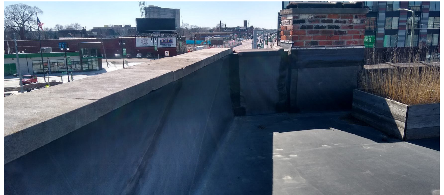
EXISTING PARAPET (LOOKING WEST)
