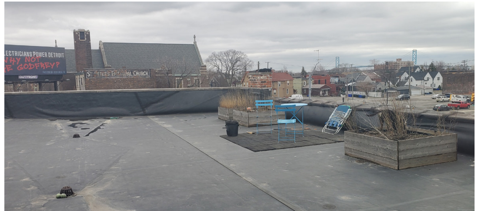
BACK OF MICHIGAN AVE.-FACING PARAPET
