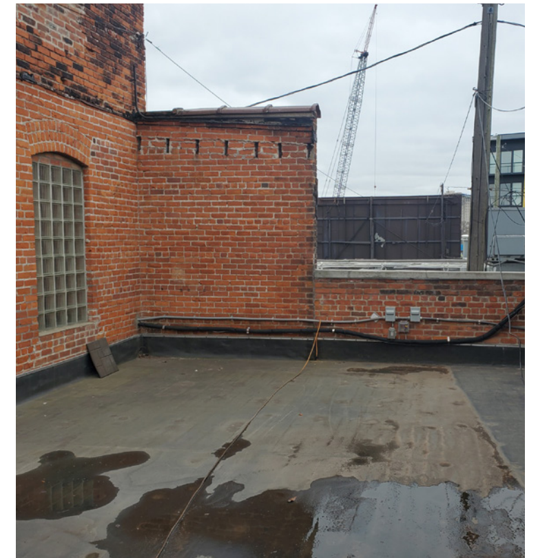
EXISTING SECOND/THIRD LEVEL NORTH FACADE (LOOKING WEST)
