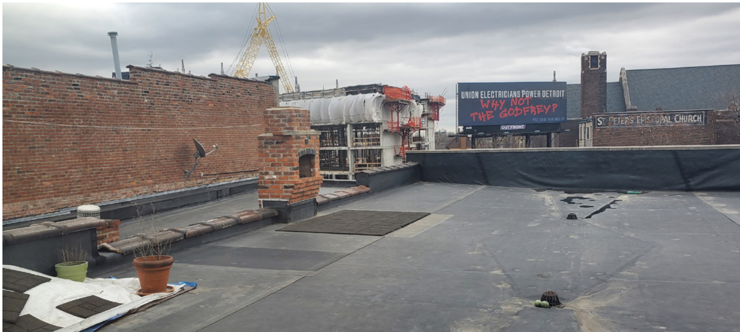
BACK OF MICHIGAN AVE.-FACING PARAPET
