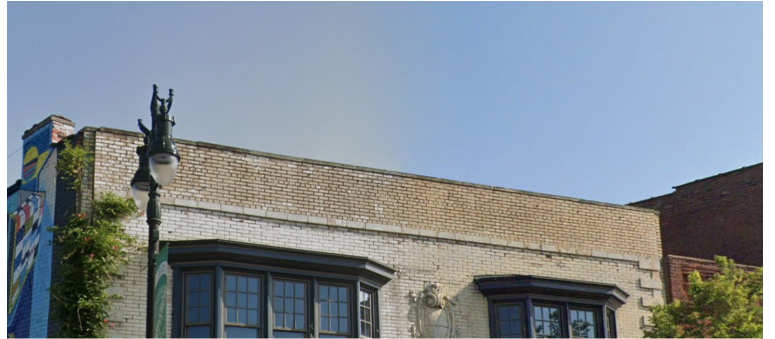
FRONT OF MICHIGAN AVE.-FACING PARAPET
