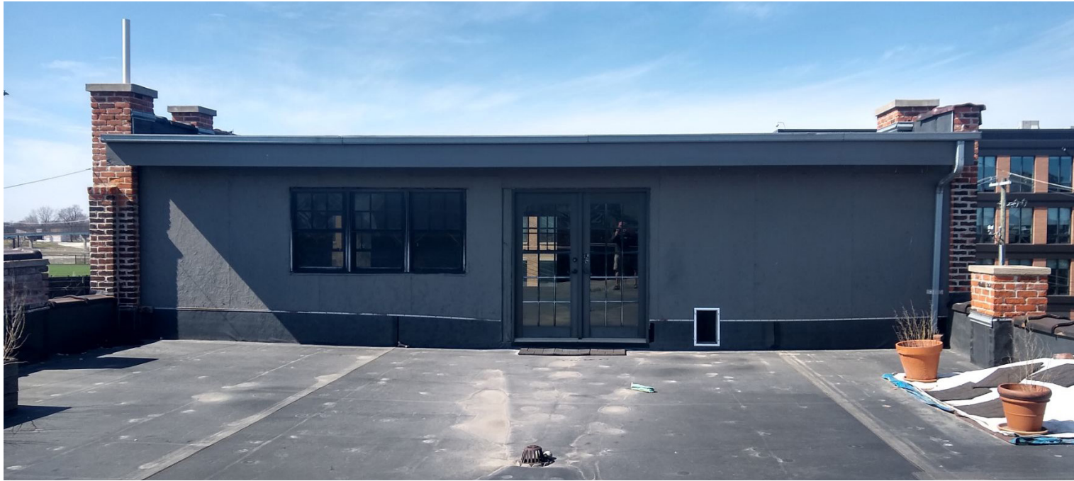
EXISTING THIRD LEVEL SOUTH FACADE
