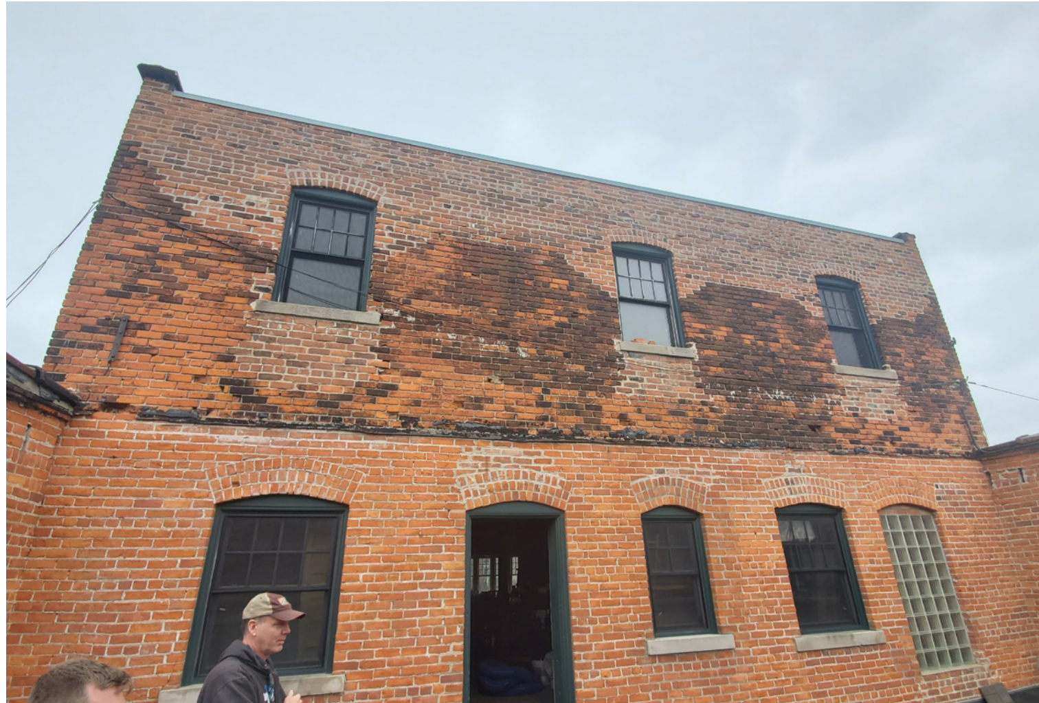
EXISTING SECOND/THIRD LEVEL NORTH FACADE
