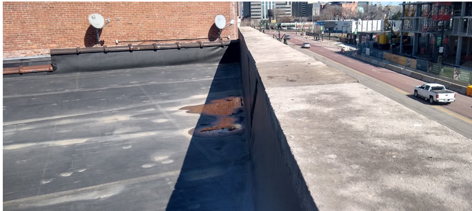
EXISTING PARAPET (LOOKING EAST)
