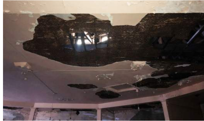
FIGURE A2.14 DETERIORATING INTERIOR PLASTER BELOW THE HEPTAGONAL ROOF STRUCTURE; SUN LIGHT IS VISIBLE THROUGH THE HOLE IN THE ROOF ABOVE
