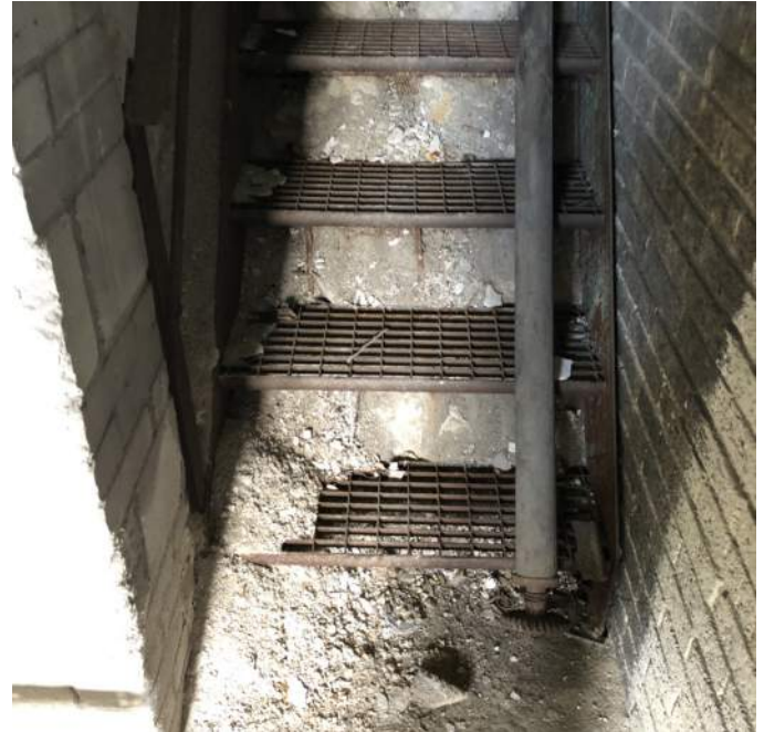
FIGURE INT 1.3 INTERIOR PLASTER HAS CRUMBLLED FROM THE WALLS, CEILING AND STRINGER BEHIND THE STAIR (LEADS TO THE ROOFTOP EXIT)
