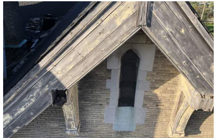
FIGURE A4.24 WEATHER AND FADED FASCIA BOARDS; DECAYED HOLLOWED WOODEN SUPPORT BRACKET
