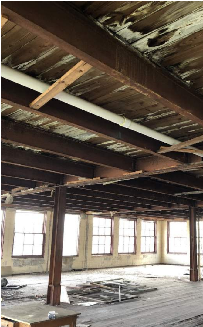
FIGURE INT 1.2 WATER STAINED AND LOOSE WOOD DECKING; OXIDIZED STRUCTURAL BEAM AND COLUMNS; VARIOUS DEBRIS; AT 1917 ADDITION INTERIORS
