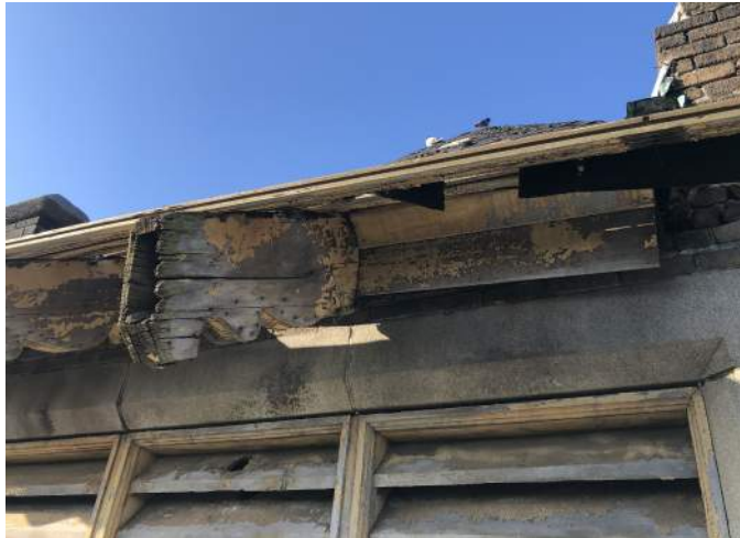
FIGURE A3.8 ROTTED DECORATIVE WOOD RAFTER TAIL AND DETACHING FRIEZE BOARD TRIM
