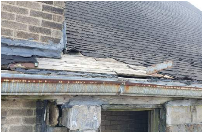
FIGURE A4.9 WEATHERED FASCIA BOARD; DECAYED WOOD DECKING; CURLLED, FRAYED AND MISSING ASPHALT SHINGLES ABOVE ROOFTOP STAIR ENTRY.
