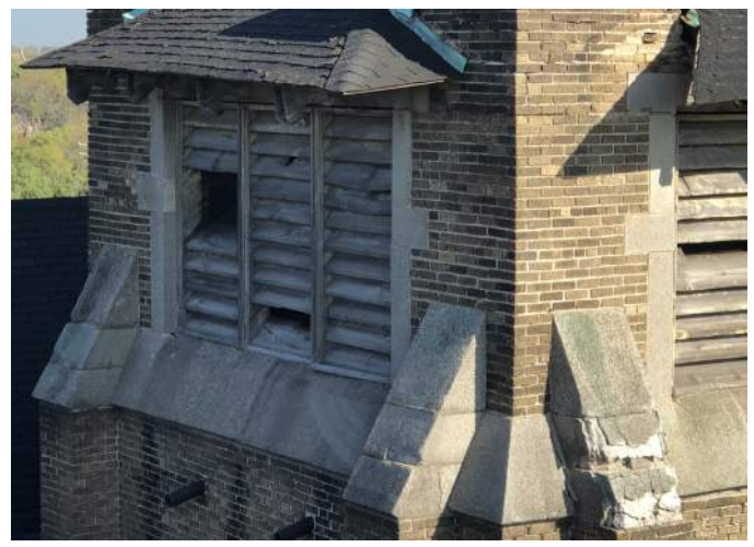
FIGURE A3.12 SOUTH WEST ELEVATION OF BELL TOWER; CRUMBLING STONE AT THE COLUMN CAP; BRICK MOVEMENT DIRECTLY UNDER THE ROOF
