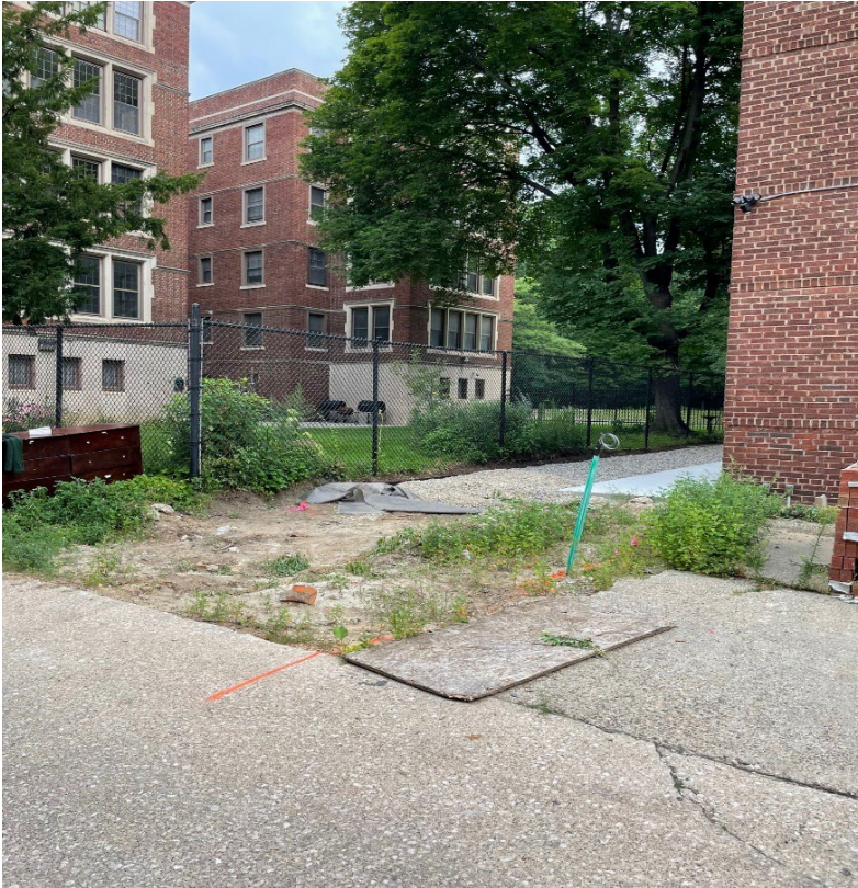
Photo 2: View of Right Center Area from Alley
