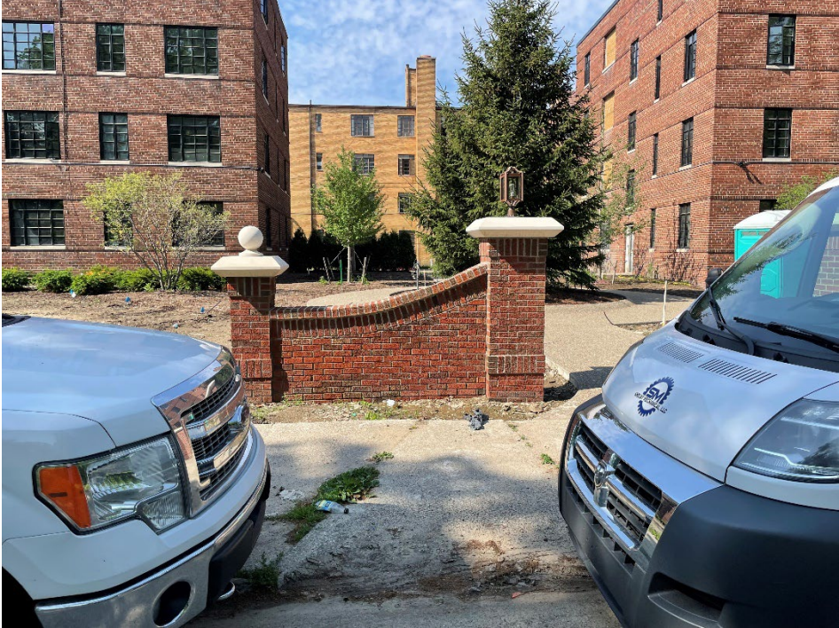
Photo 7: View of Central Courtyard from Street
