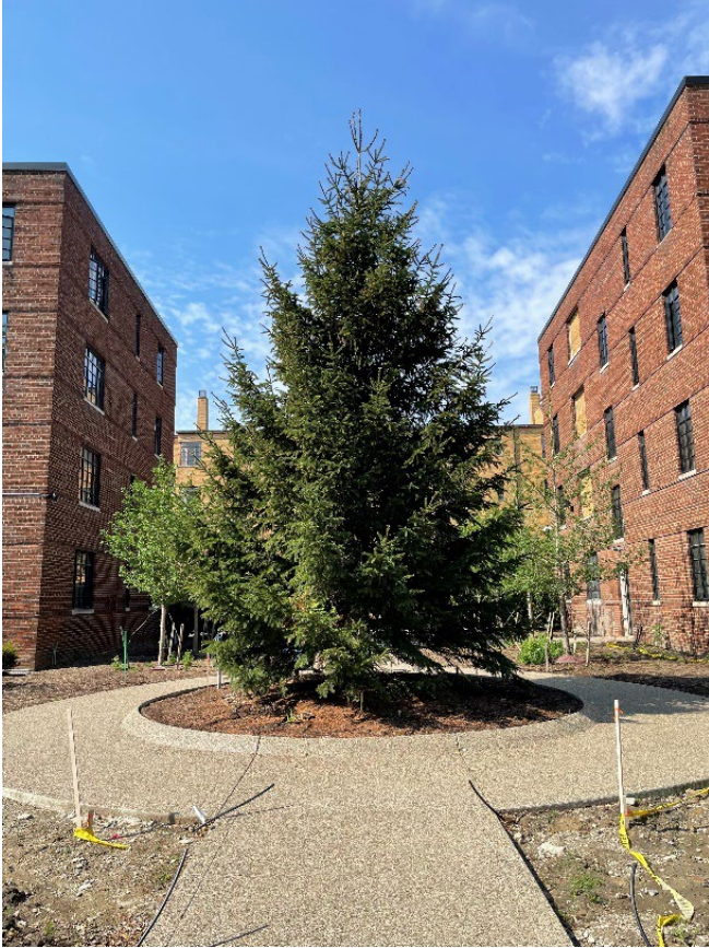
Photo 6: View of Central Courtyard between 885/931
