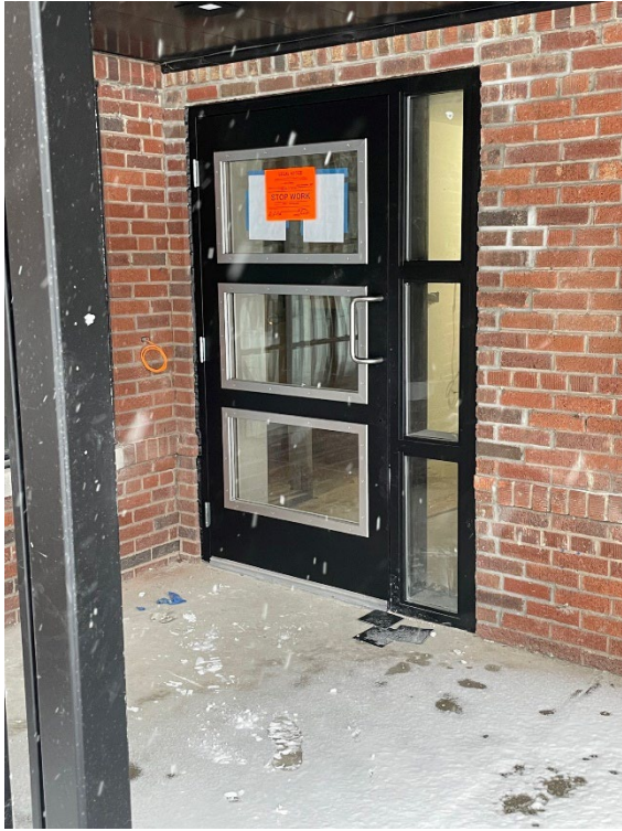
Photo 3: View of 885 Covington Entry Door
