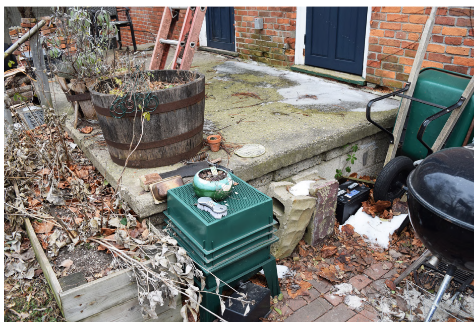
SIDE PORCH BASE AND STEPS TO BE REMOVED
