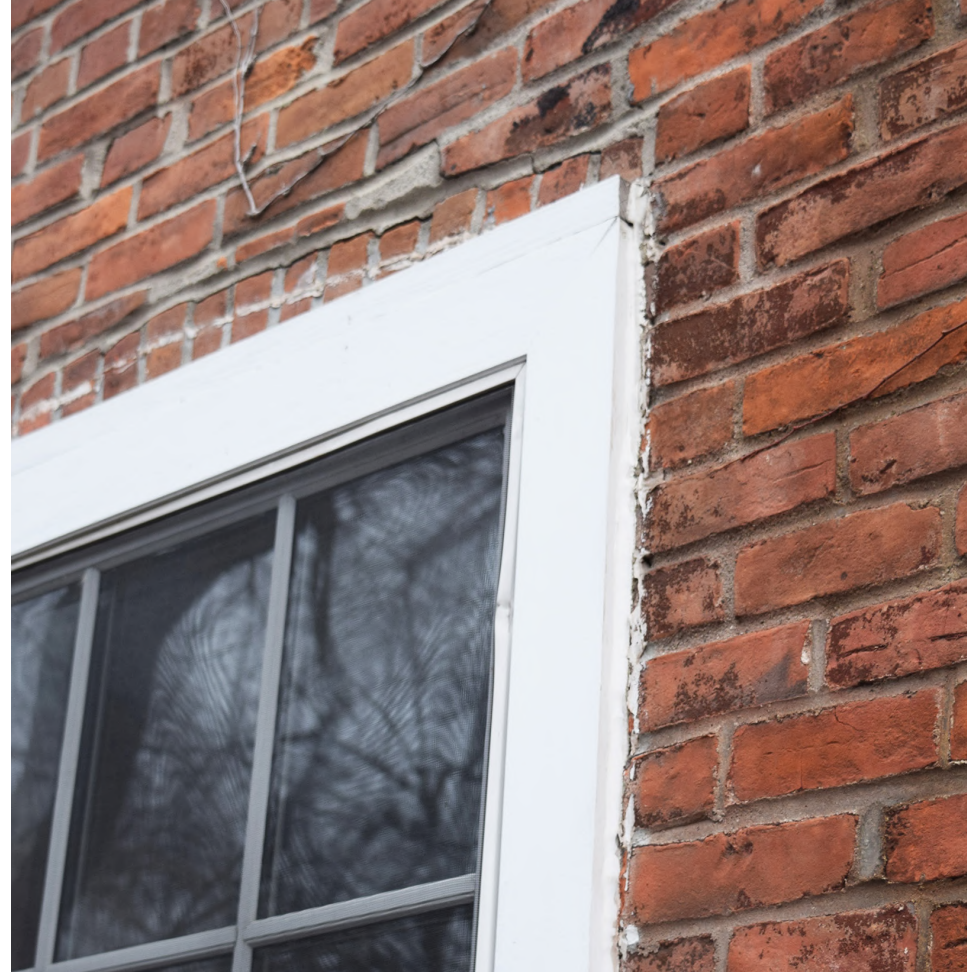
TOP MIDDLE TYPICAL WINDOW HEAD DETAIL AT ARCHED OPENINGS. ALL WINDOWS (INSTALLED DURING 1992 RENOVATION) EXHIBIT IMPROPER INSTALLATION IN MASONRY OPENINGS. CAULK SEALANT HAS DETERIORATED AND REGULARLY LEAKS.
