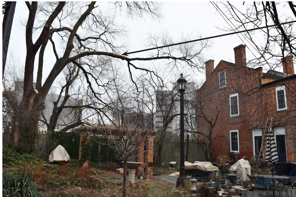
DEAD LIMBS OF LARGE TREE AT SIDE YARD TO BE REMOVED
