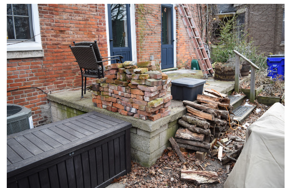
SIDE PORCH BASE AND STEPS TO BE REMOVED
