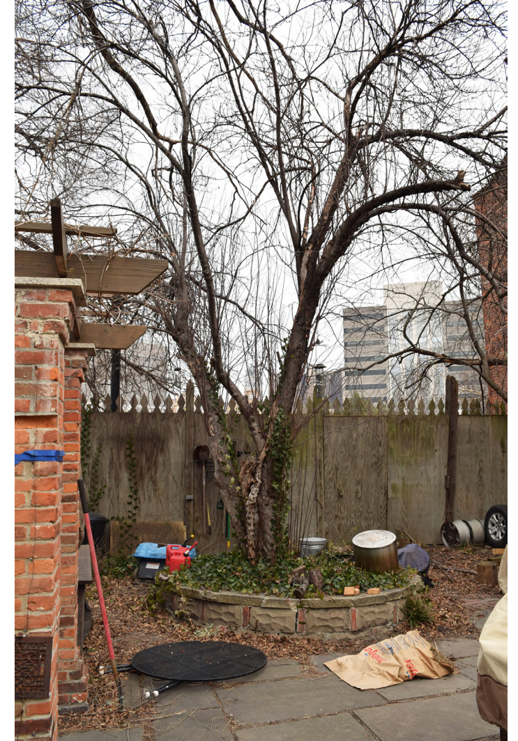
APPLE TREE AND CMU PLANTING BED IN FOOTPRINT OF ADDITION AT SIDE YARD TO BE REMOVED
