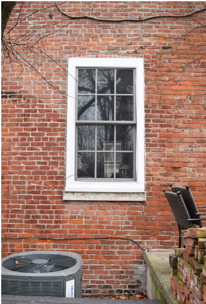
2. WINDOW TO BE REMOVED AND OPENING INFILLED- AREA WILL BE ENCLOSED BY ADDITION WITH FIRE- RATED FURRED WALL
