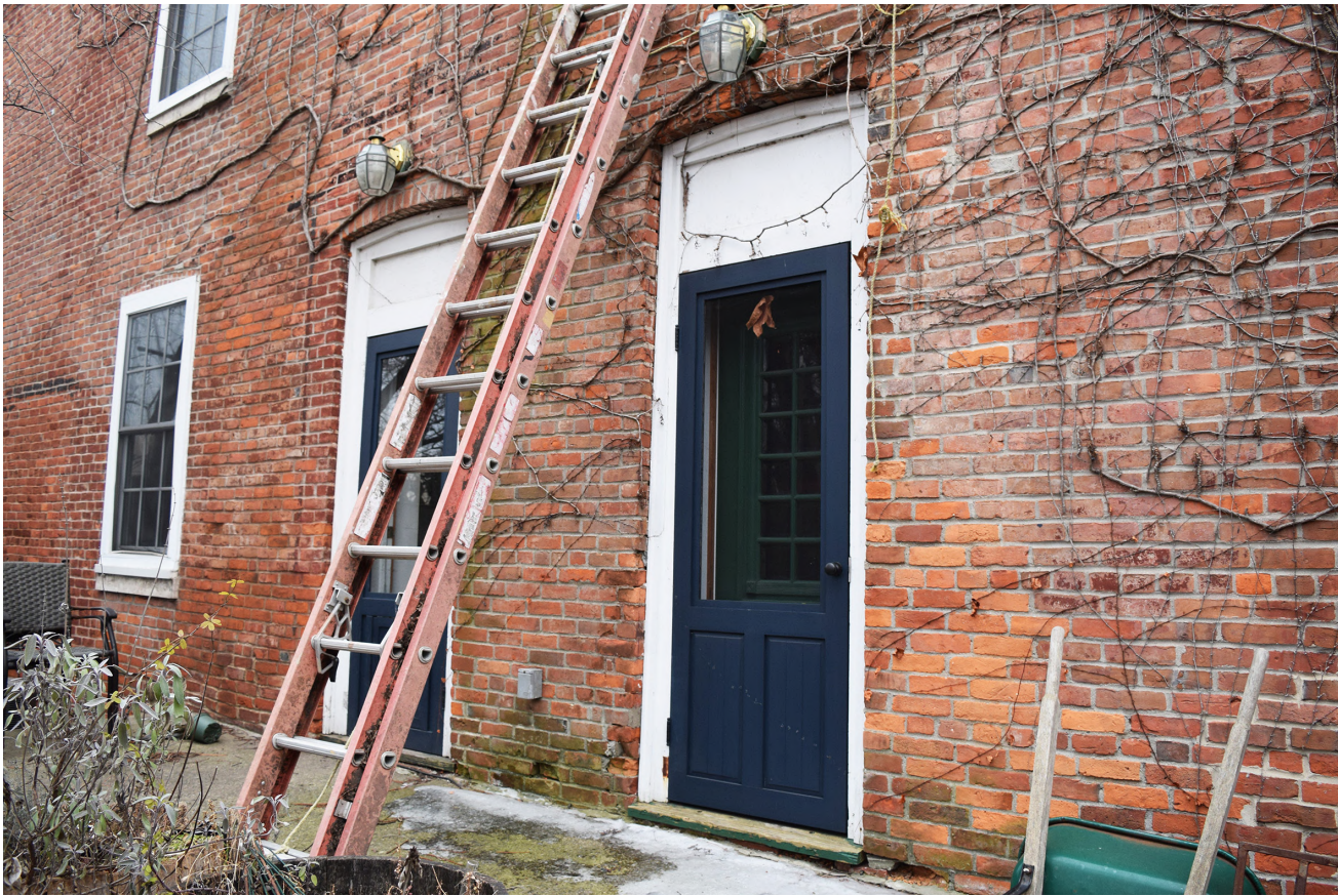
2. WINDOW TO BE REMOVED AND OPENING INFILLED- AREA WILL BE ENCLOSED BY ADDITION WITH FIRE- RATED FURRED WALL
