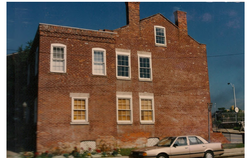
RENOVATION NEAR COMPLETION
