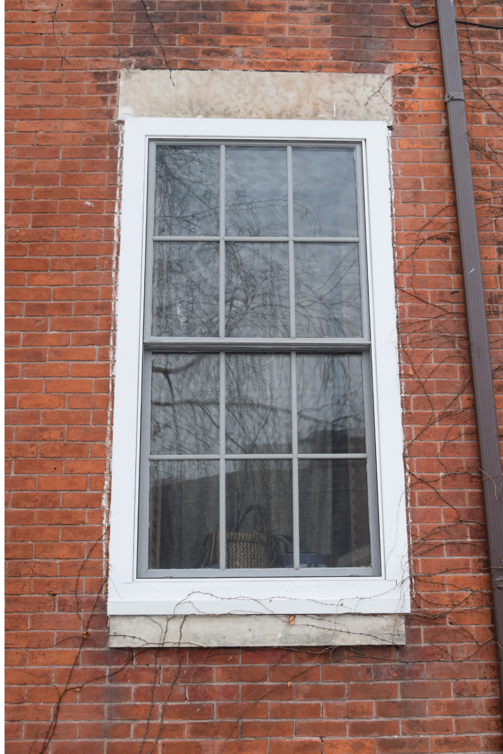
TOP MIDDLE TYPICAL WINDOW HEAD DETAIL AT ARCHED OPENINGS. ALL WINDOWS (INSTALLED DURING 1992 RENOVATION) EXHIBIT IMPROPER INSTALLATION IN MASONRY OPENINGS. CAULK SEALANT HAS DETERIORATED AND REGULARLY LEAKS.
