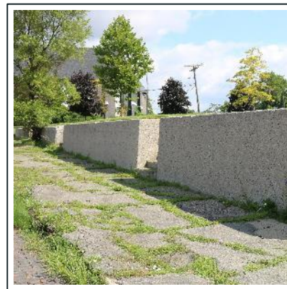
17 th Street Retaining Wall (1914)
