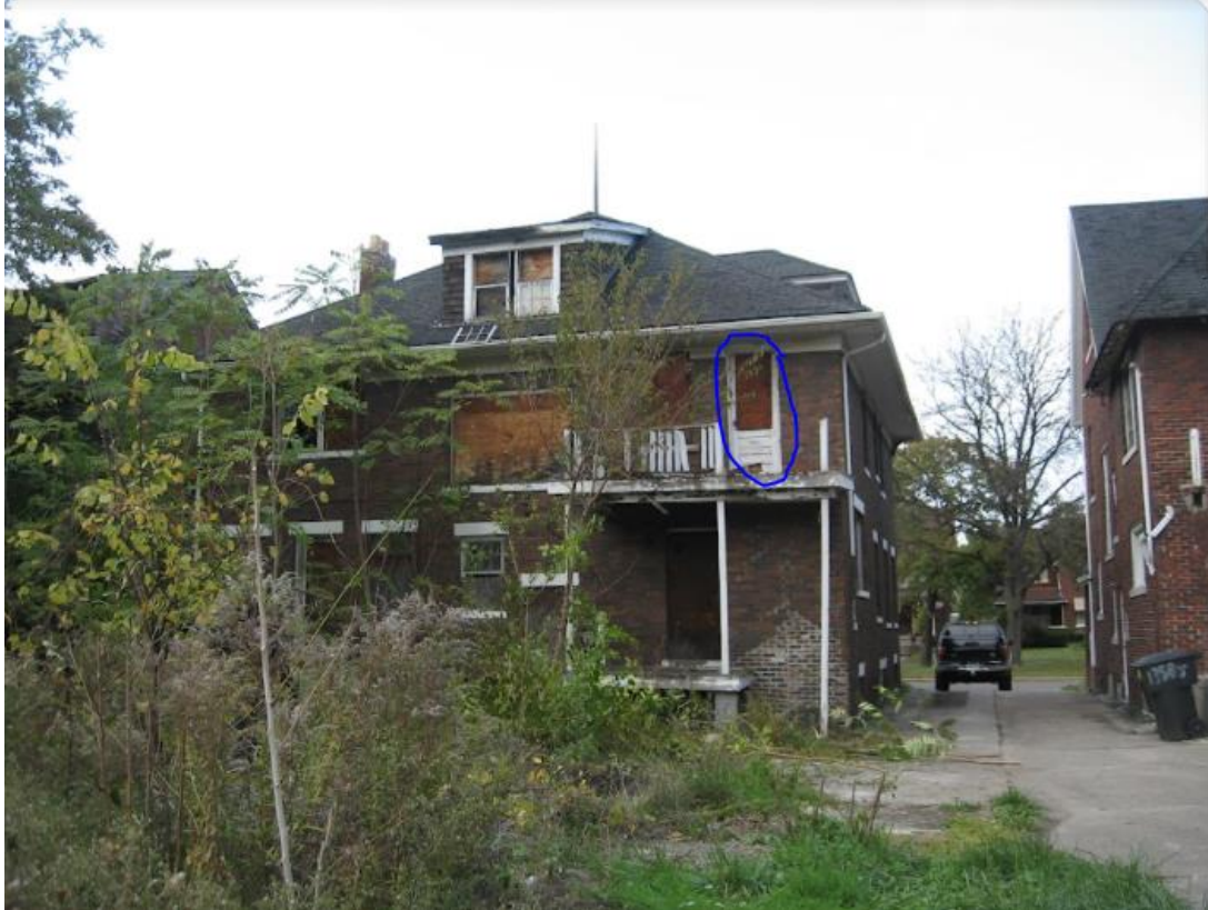
Original home as purchased (NOV 2014)– Rear. Replace upper rear exterior door
