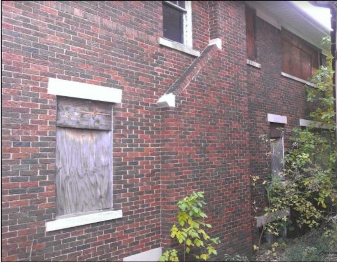
Original home as purchased (NOV 2014)– Opposite Side
