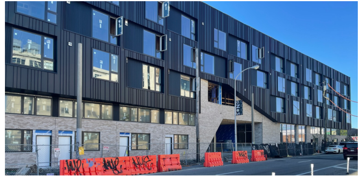
STANDING SEAM PROFILE IDENTICAL TO CMG PRODUCT VARIABLE WIDTHS (16" TO 8") - NO STIFFENING RIBS SONO, PHILADELPHIA (IN PROGRESS)
