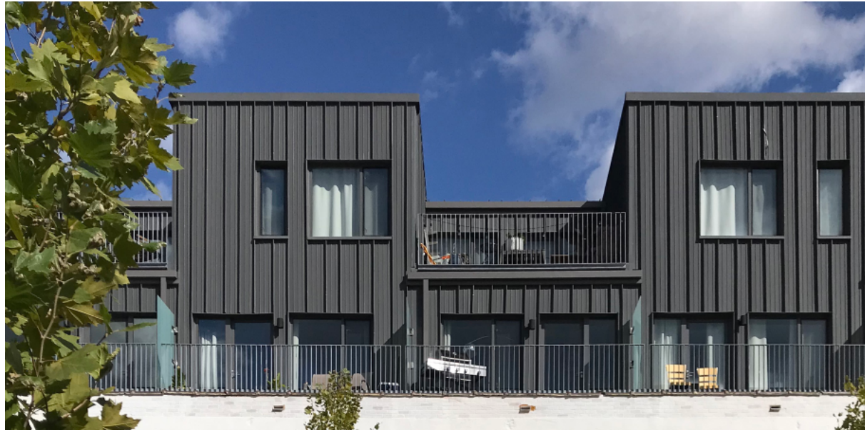
KALZIP VARIABLE WIDTHS - WITH STIFFENING RIBS 644 SELDEN, DETROIT
