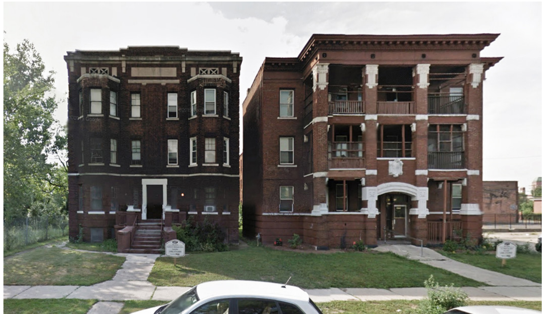
ADJACENT BUILDINGS TO THE WEST
