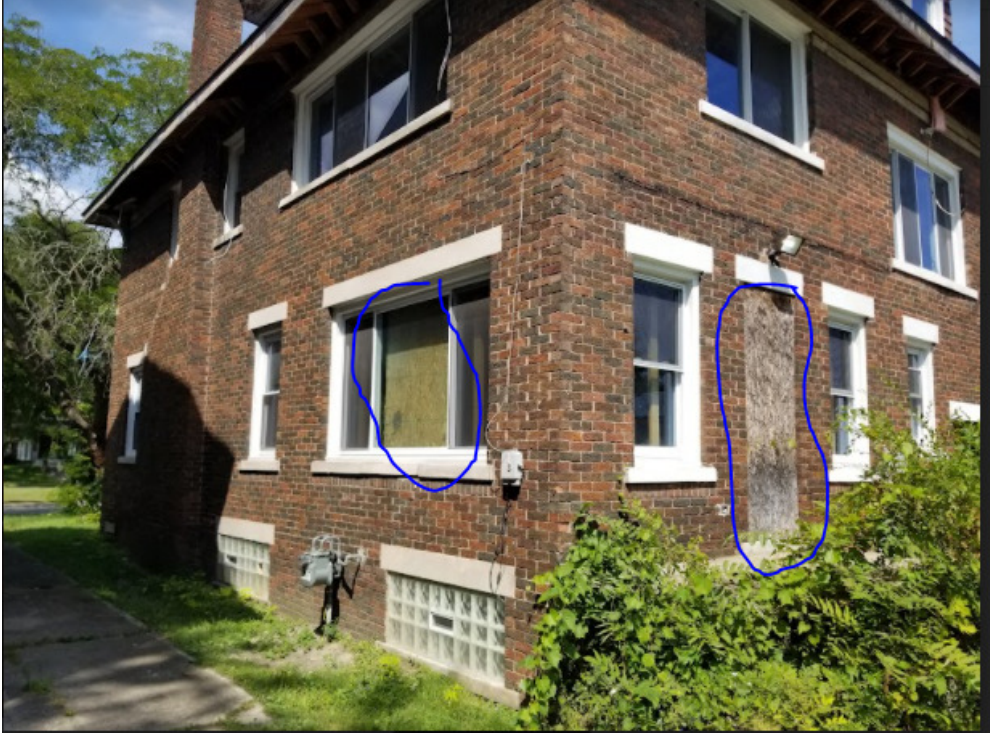
Current State – Windows replaced side window covered to prevent vandalism
