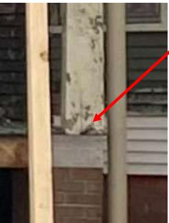
Here you can see the columns are leaning and rotting. There are no base for the columns, so they are not attached to the porch. The center column on the south elevation is not connected to the roof.
