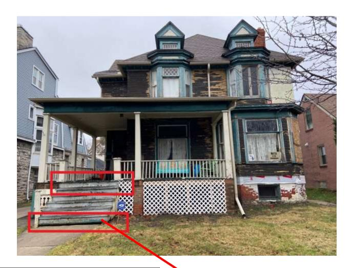
You can see from the pictures the stairs are not to code missing handrails, risers at different heights, bricks use to level the stairs.
