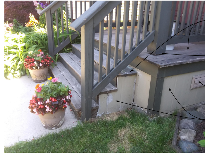
North (Front) Porch: Existing wood porch floor and steps require repair, sanding and clear waterproof coating. Stair risers to be repainted. Plywood siding to be removed and replaced with new cedar vee siding. Column base trim to be reconstructed.
