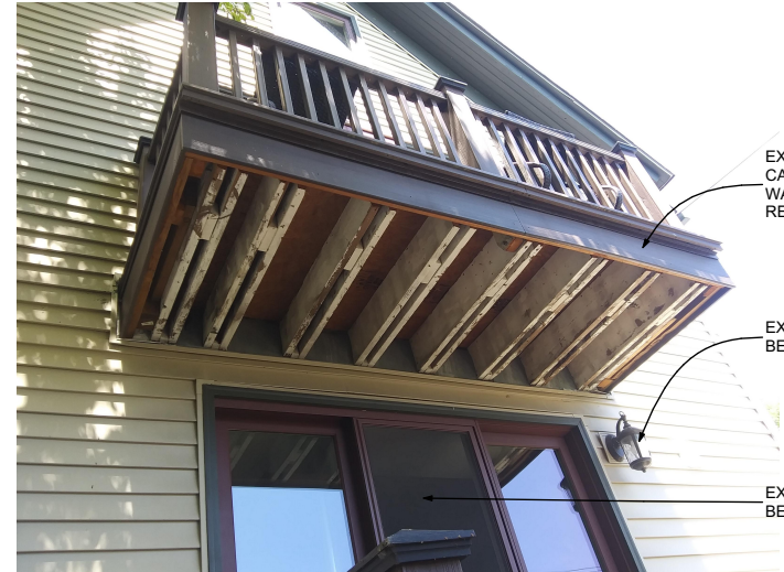
South Elevation: Second floor cantilevered walkout to be removed. This walkout is accessed from the second floor master bedroom. The walkout is a recent addition and the deck and railing systems are clad with plastic composite lumber. The recently-added rear porch light shown in this photo will be removed and replaced with a flush-mount ceiling light when the new rear porch is constructed.
