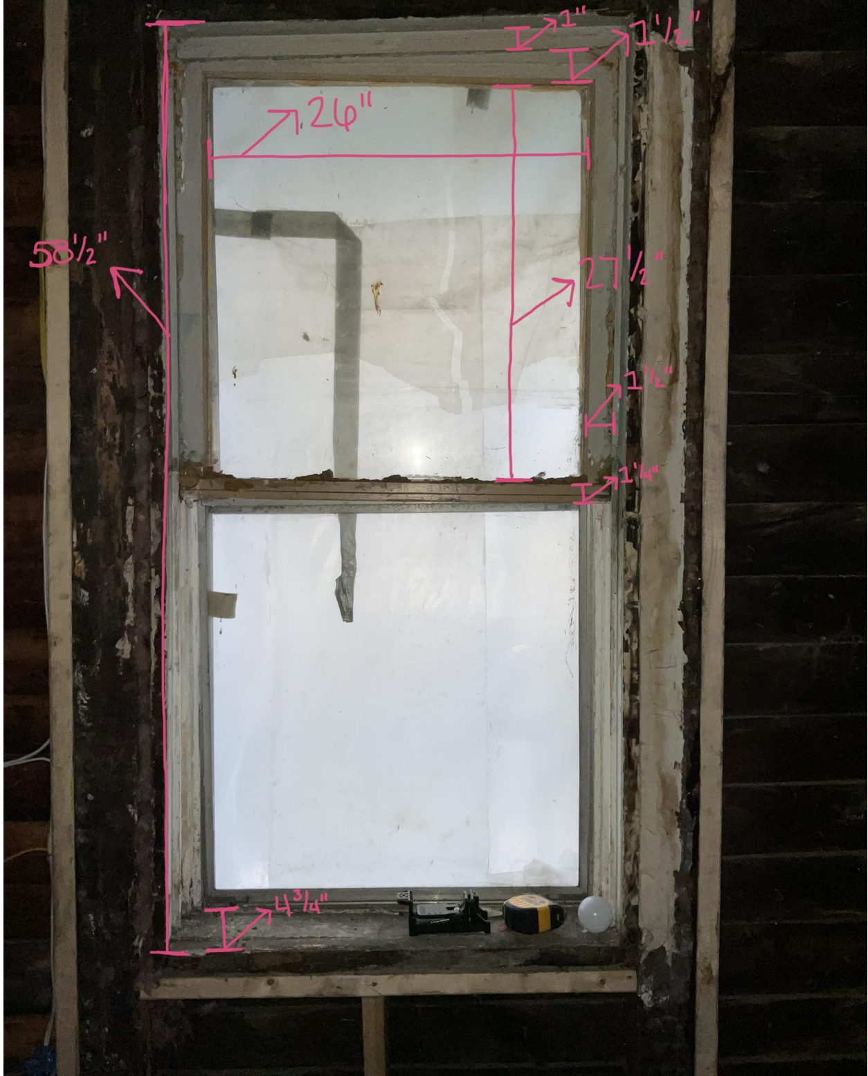
LIVING ROOM x2 (BOTTOM WINDOWS AT FRONT OF HOUSE)
