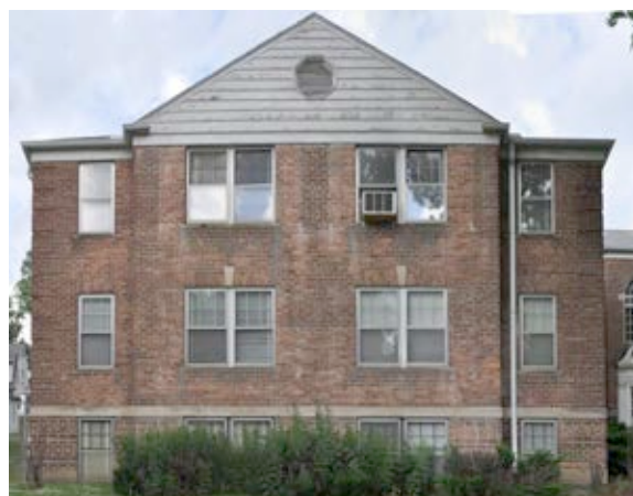
East Elevation - Northern Facade
