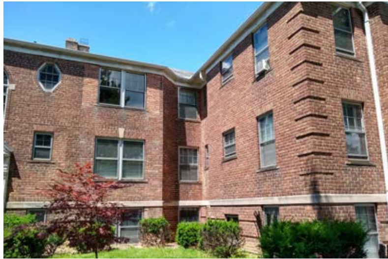
Courtyard East & North Elevation
