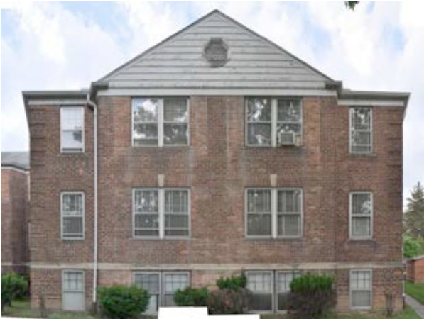
East Elevation - Southern Facade
