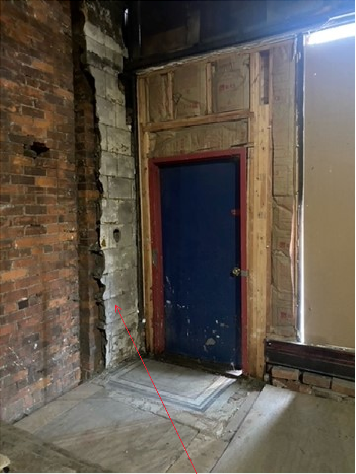
REPAIR/RESTORE SIDE WALL.
