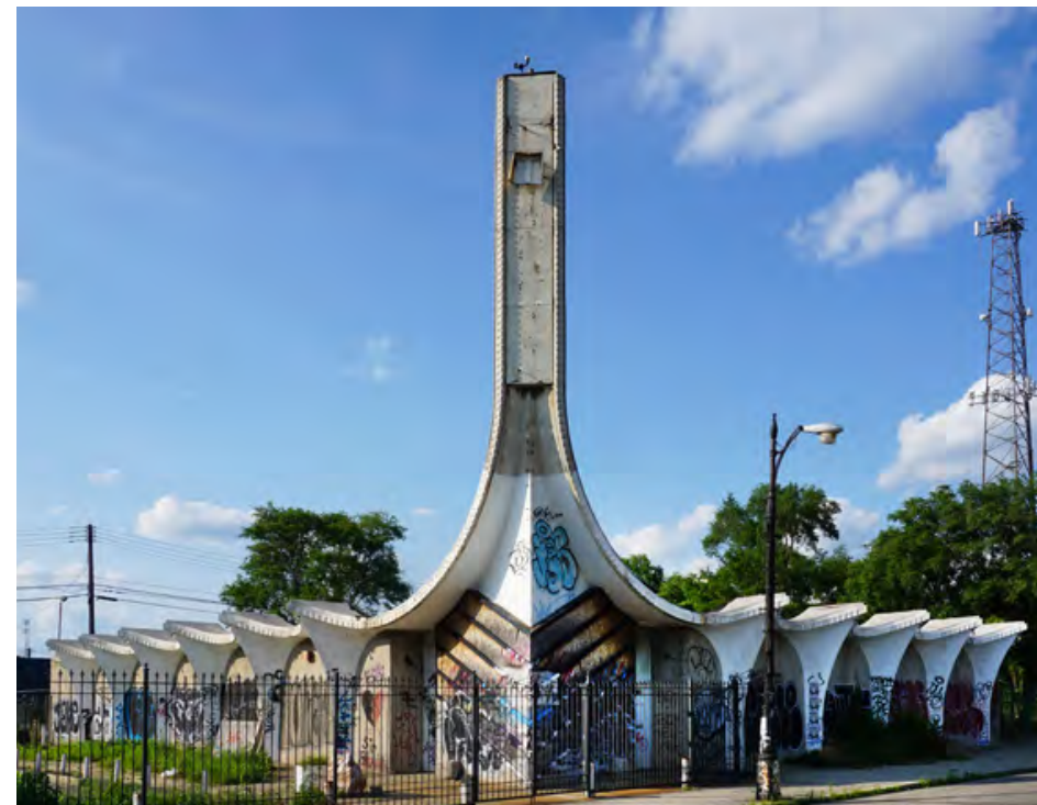
Building post 2013 with graffiti
