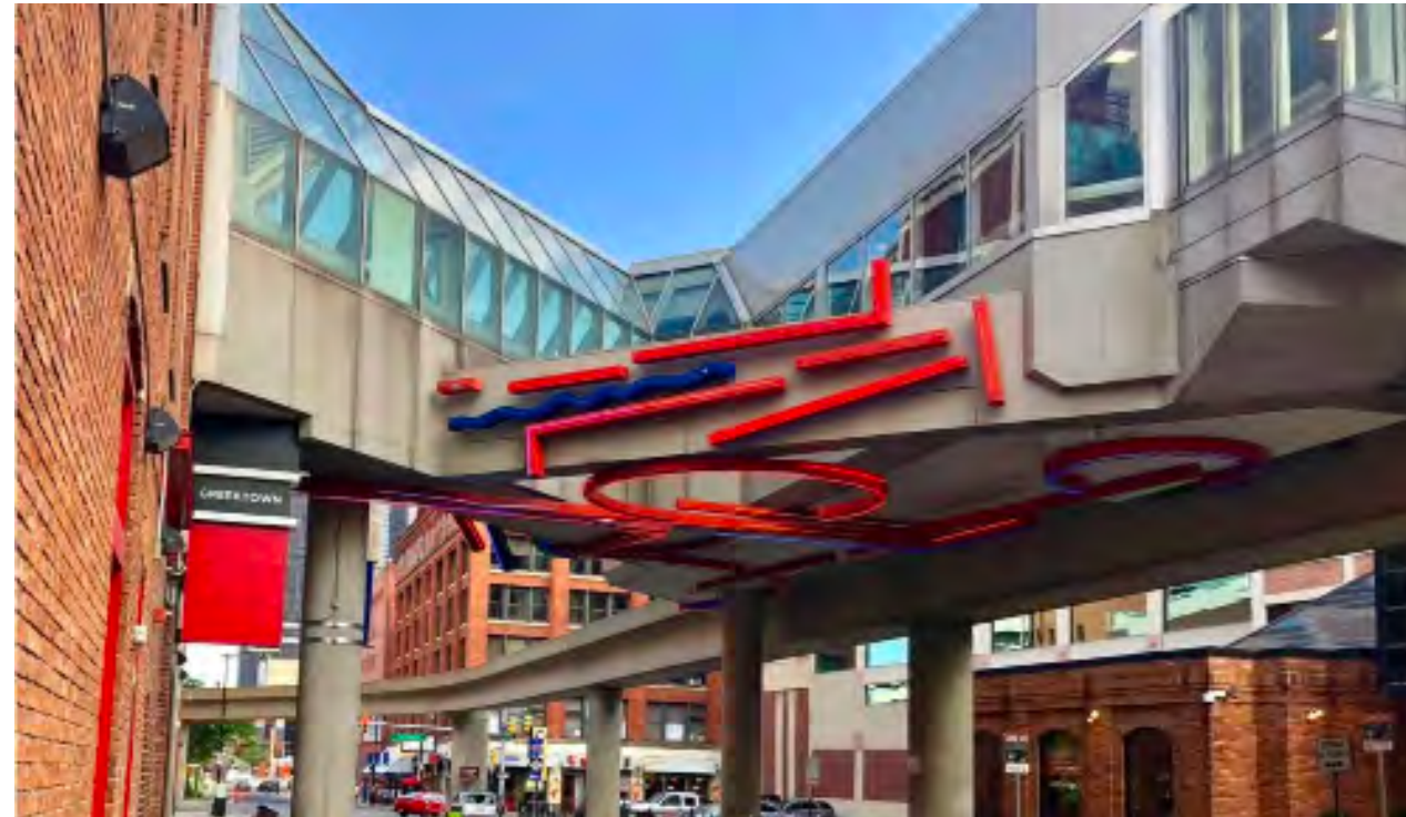
People Mover Station in Downtown Detroit
