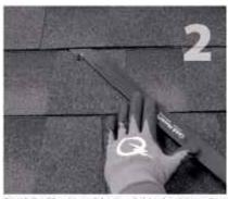
mounted. Select the courses of shingles where bar, just above placement of mount. Remove nails as required and backfill holes with aproved
