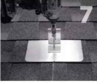
Prepare lag bolt or structural screw with sealing You are now ready for the rack of your choice. washer. Using a 1/2-inch socket on an impact gun, drive prepared lag bolt through L-foot until L-foot can no longer easily rotate. DO NOT over-torque. NOTE: Structural screw can be driven with T-30 hex
