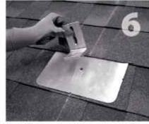
Place L-foot onto elevated flute and rotate L-foot to desired orientation.
