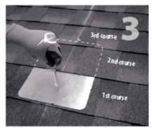
up so top edge of flashing is at least 44\* higher than the butt-edge of the 3rd course and lower sealant. See "Proper Flashing Placement" on next flashing edge is above the butt-edge of 1st course. Mark center for drilling.
