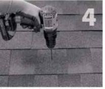
1/4" bit (ST) for attaching with the structural screw. compatible with roofing materials. Drill pilot hole into roof and rafter, taking care to drill square to the roof. Do not use mount as a drill guide. Drill a 2" deep hole into rafter.
