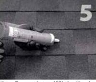
If attaching with lag bolt use a 1/22\* bit (Lag). Use a Clean off any sawdust, and fill hole with sealant
