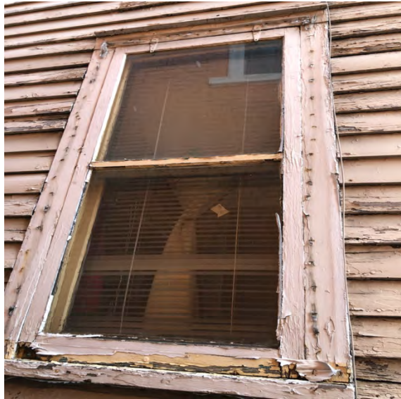
Deteriorated Window
