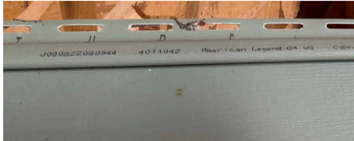
Existing Vinyl Siding: American Legend - Double 4" Clapboard - Cypress
