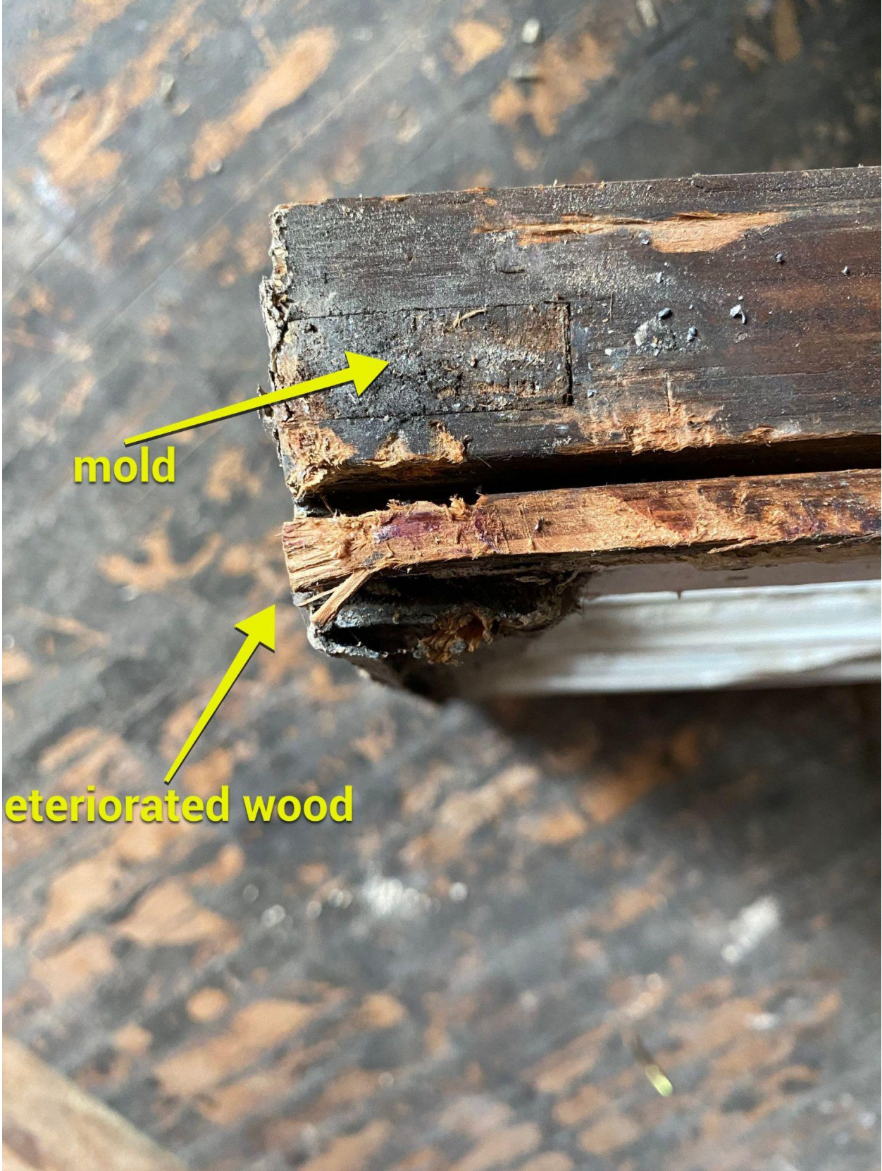
Window 4, 9/1 divided light South Elevation - Right Sash
