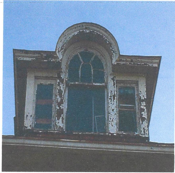
Wall A Roof Dormer
