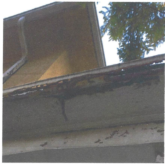
Damaged Gutter
