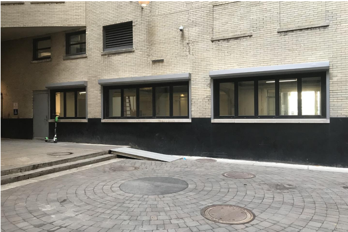
Figure 2: Western Courtyard, Looking North. 6/3/21
