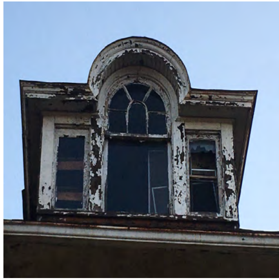
Wall A Roof Dormer
