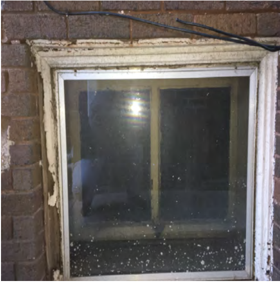
Most Cellar Windows are Covered with Storm Sashes
