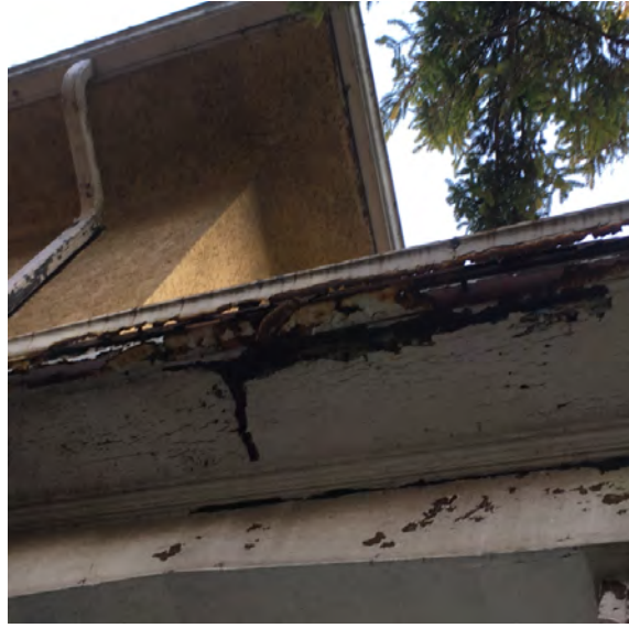
Damaged Gutter
