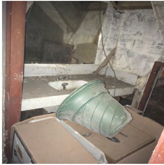
Basement Bathroom (Not In Use)
