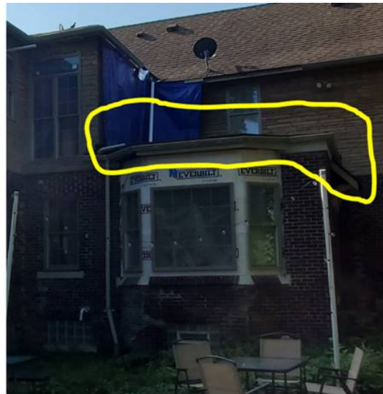
After removal – June 2021
