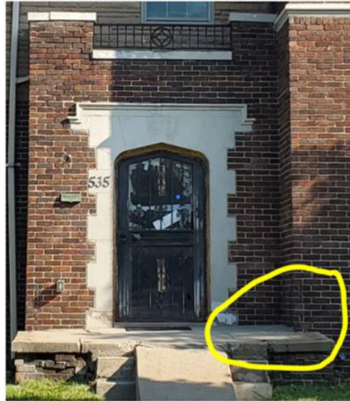
After removal – June 2021
