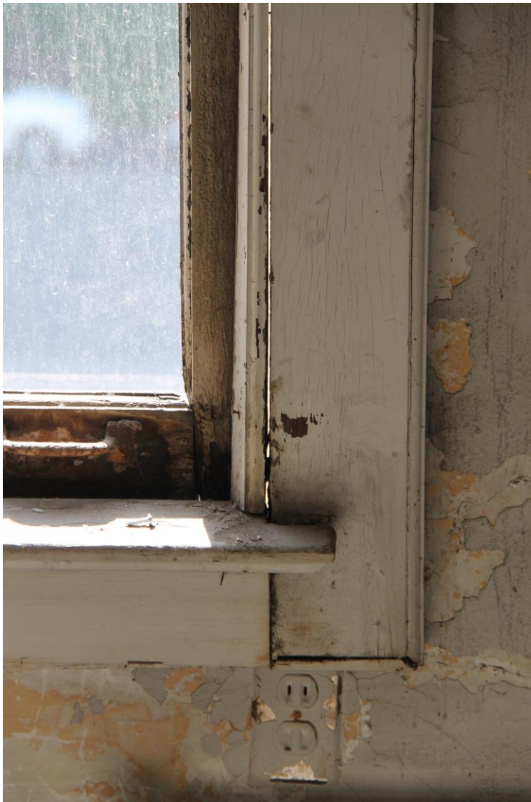
INTERIOR JAMB WITH DAYLIGHT SHOWING
