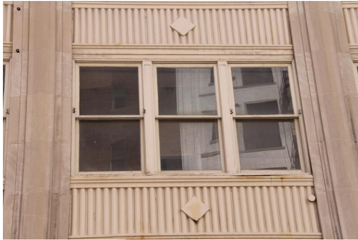
TYPICAL EXTERIOR VIEW
