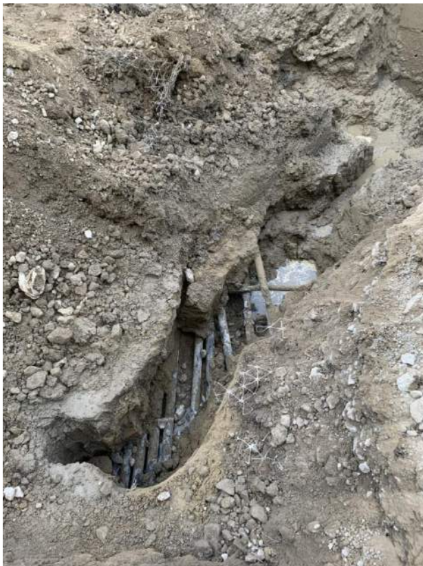
Existing geothermal is shallow and not shown in locations on plans
