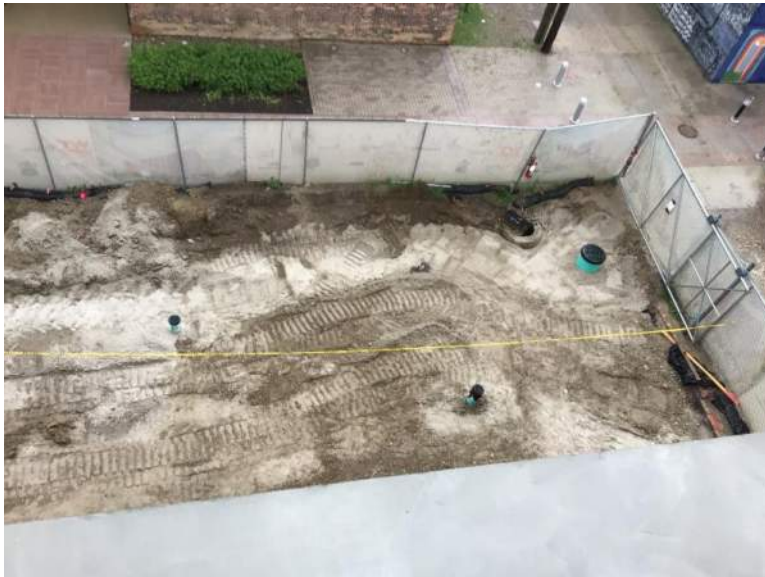
North portion of Green Alley with drainage system installed
