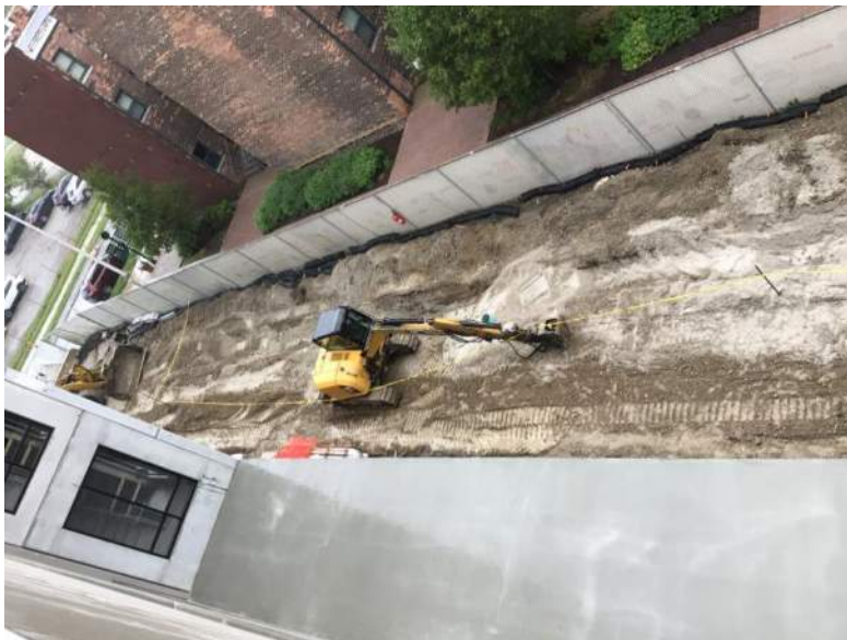
South portion of Green Alley with drainage system installed
