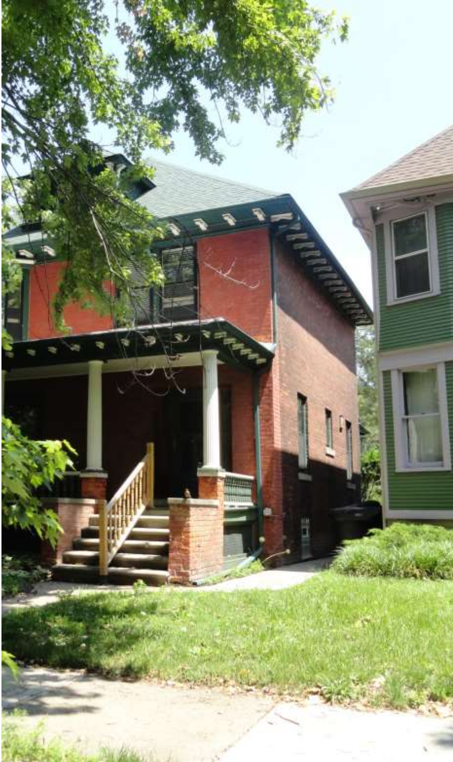
Side Elevation Facing South
