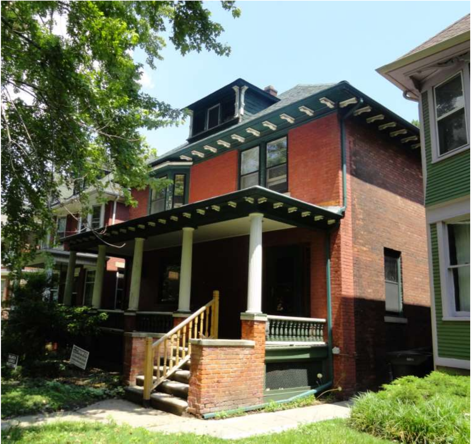
Front Façade Facing Street, West
