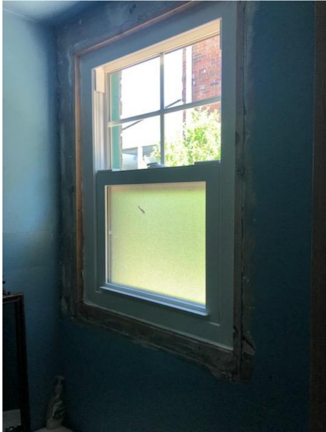
1ST FLOOR BATHROOM
