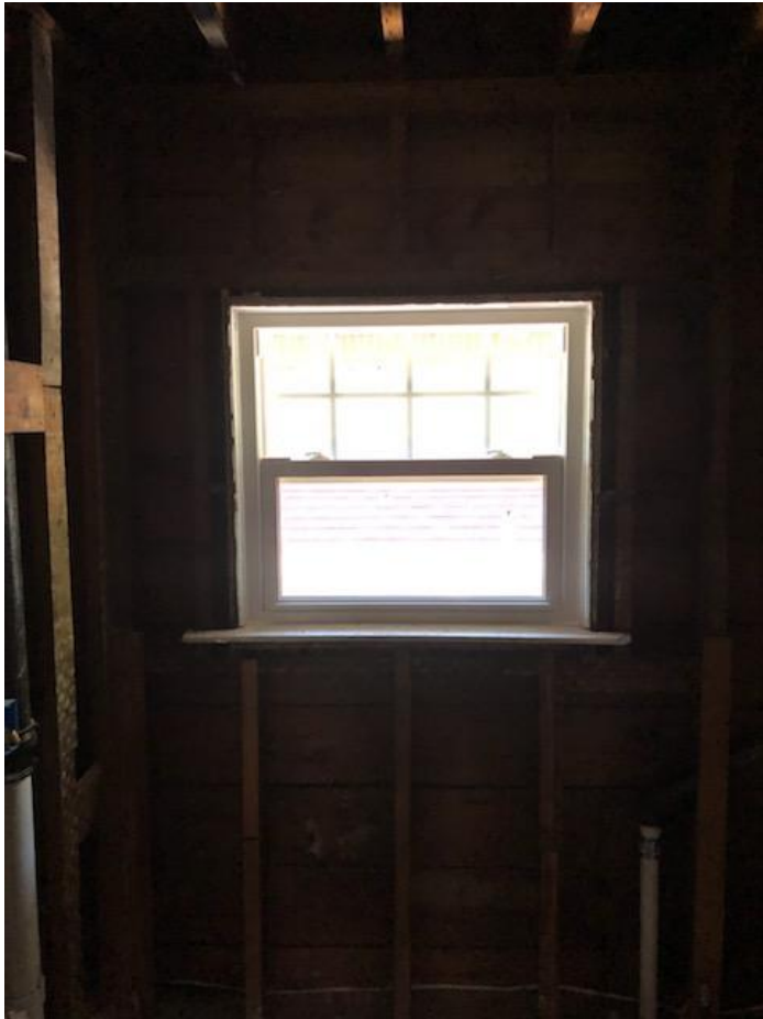
2ND FLOOR BATHROOM (SIDE)
