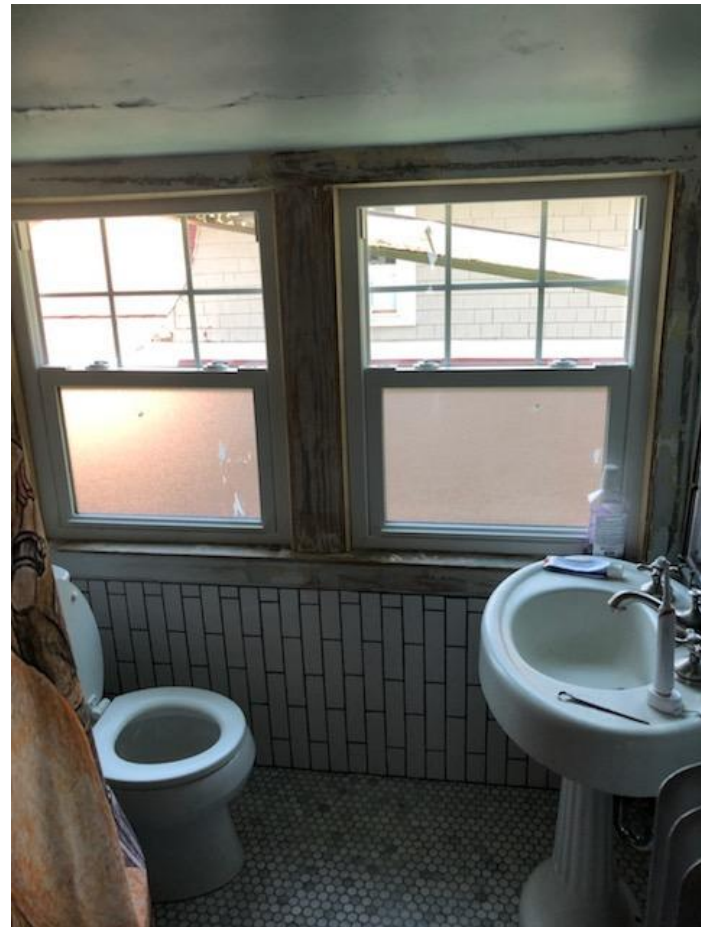
3RD FLOOR BATHROOM
