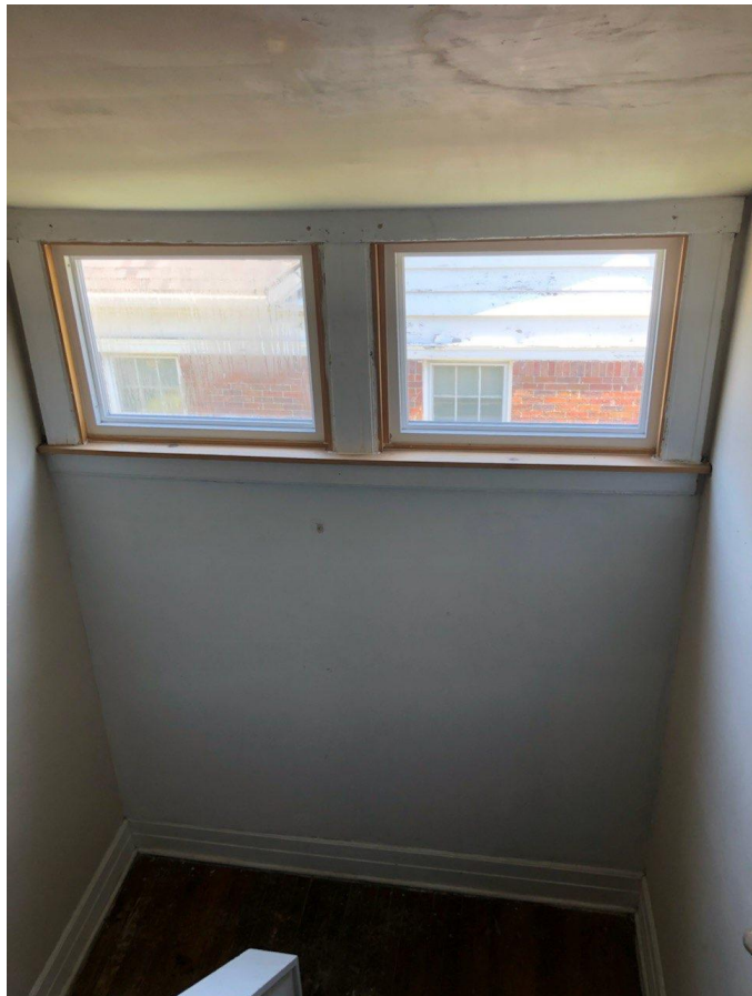
3RD FLOOR STAIRWAY
