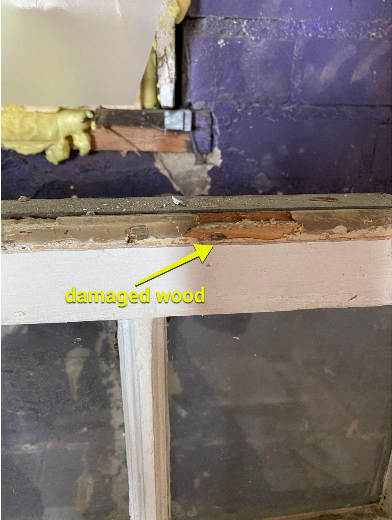
Window 9, 12/1 divided light South Elevation
