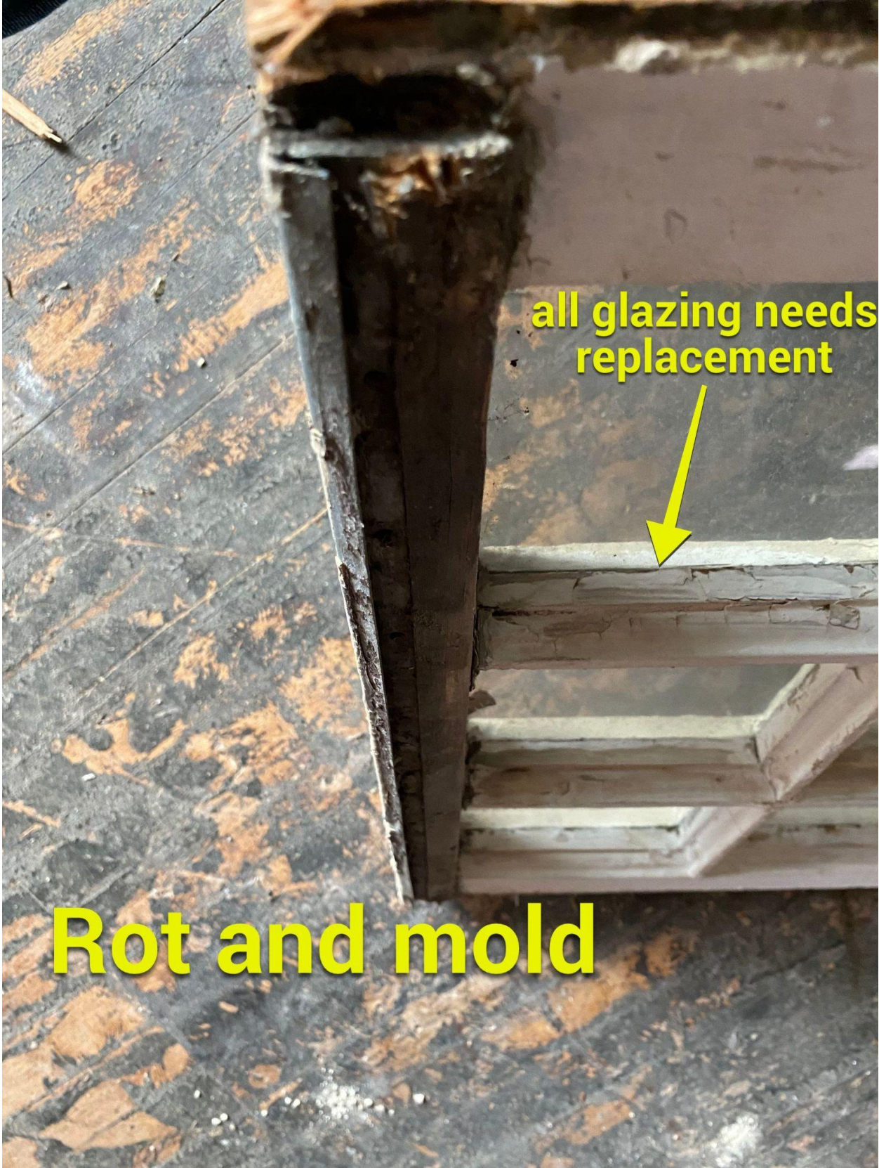
Window 5, 9/1divided light South Elevation
