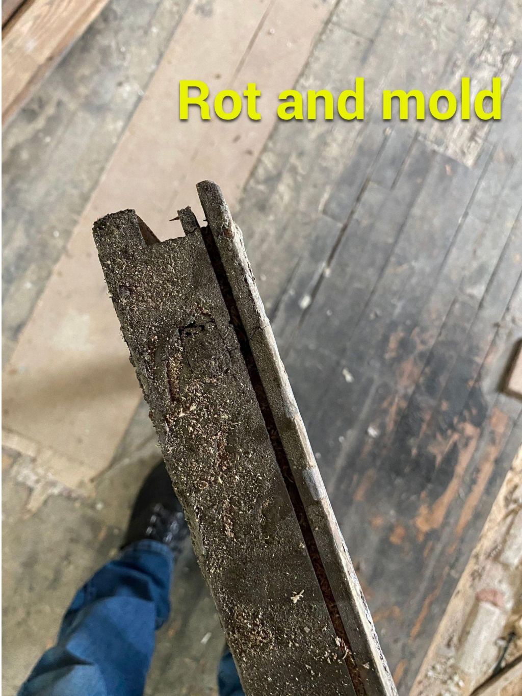
Window 3, 9/1 divided Light South Elevation - Bottom Rail
