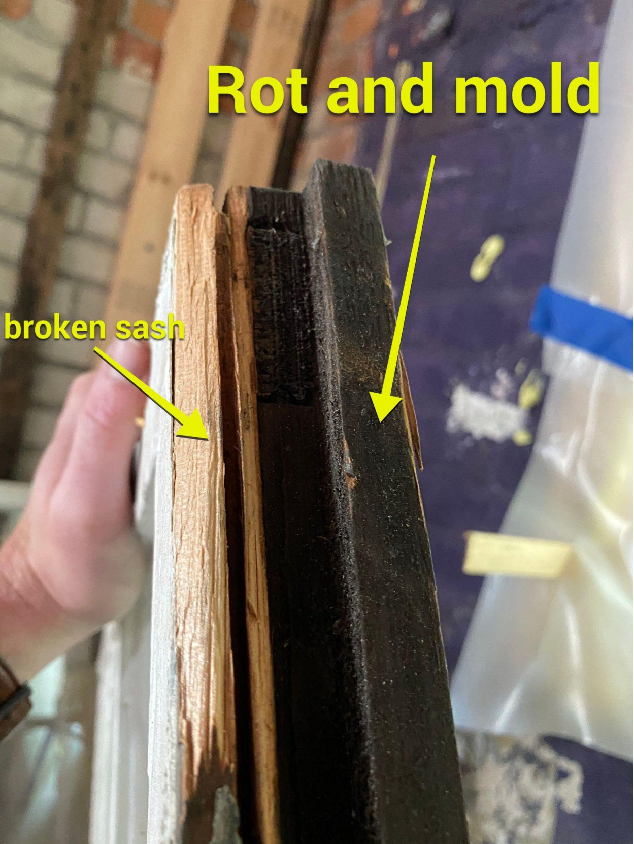
Window 7, 12/1 divided light South Elevation
